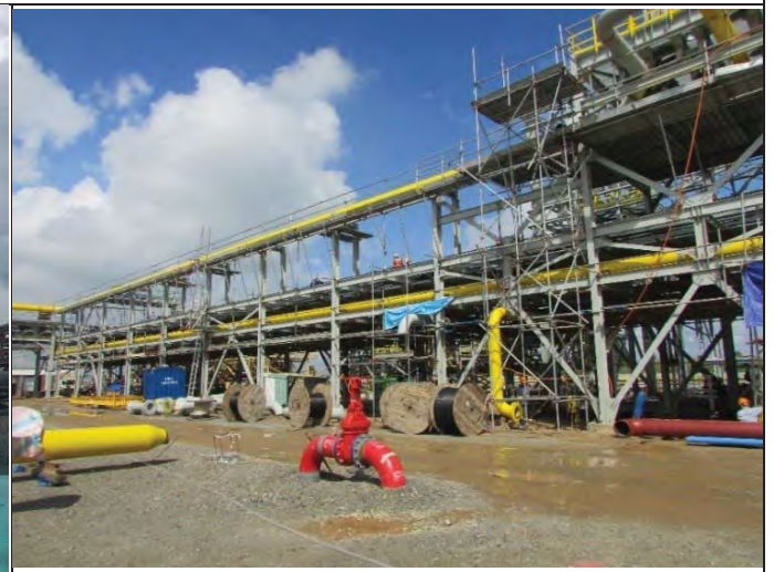
INSTALLATION OF STAINLESS STEEL PIPE FOR IDEMITSU LUBE OIL PLANT
