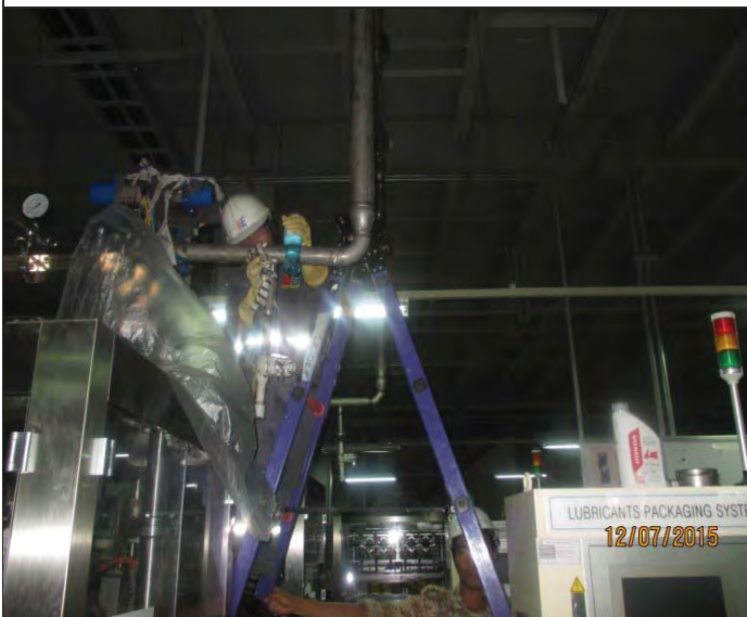
INSTALLATION OF STAINLESS STEEL PIPE FOR IDEMITSU LUBE OIL PLANT
