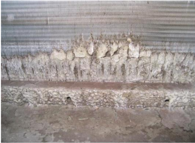
Examples of heavy microbial growth on coil and trays (Source: Opira Group)
