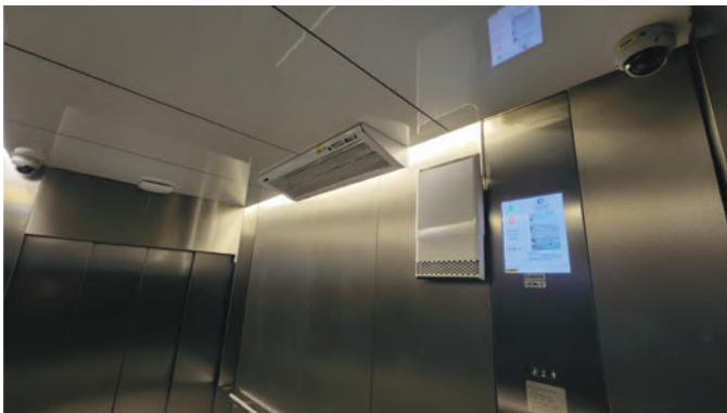
Combined air and surface disinfection installed in far north Queensland hospital service lift
