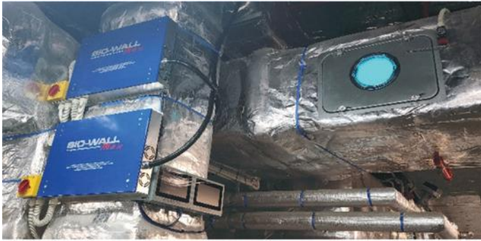
Examples of in-duct UVC 254 air disinfection installations (Source: Opira)
