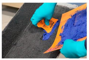
As shown in the image above, Belzona 1818 is ideally suited for patch repairs where a rapid return to service is required.
