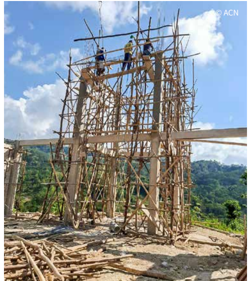
INDONESIA: Construction of chapel of Golo Popa.
