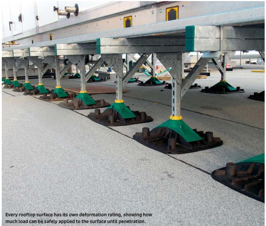
Every rooftop surface has its own deformation rating, showing how much load can be safely applied to the surface until penetration.
