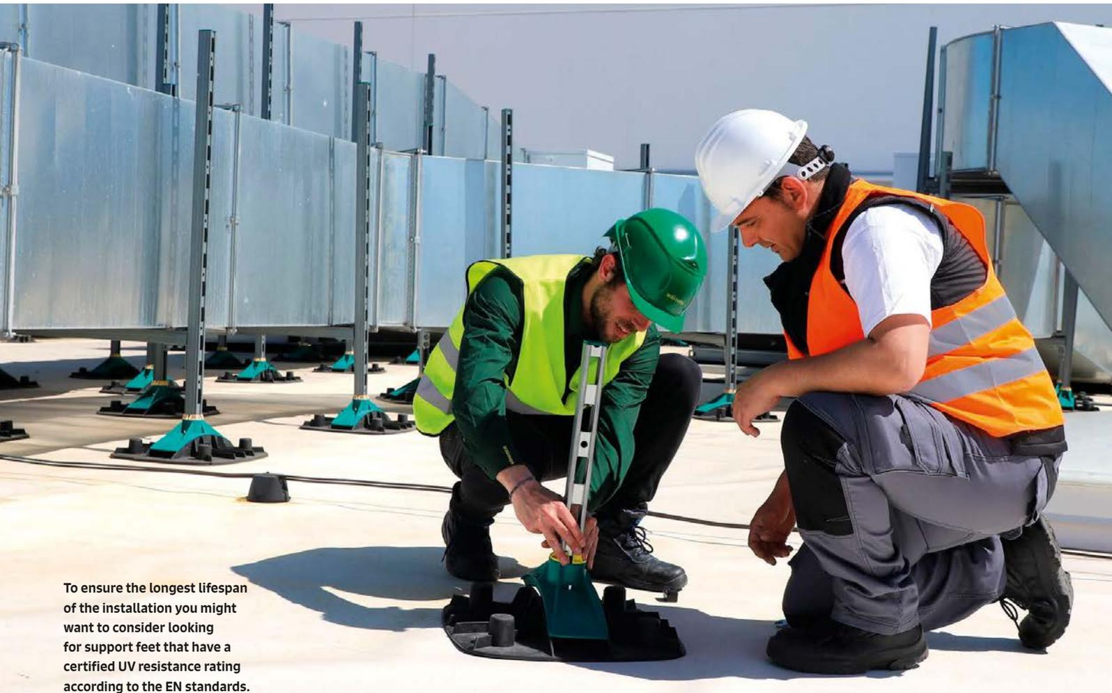
To ensure the longest lifespan of the installation you might want to consider looking for support feet that have a certified UV resistance rating according to the EN standards.
