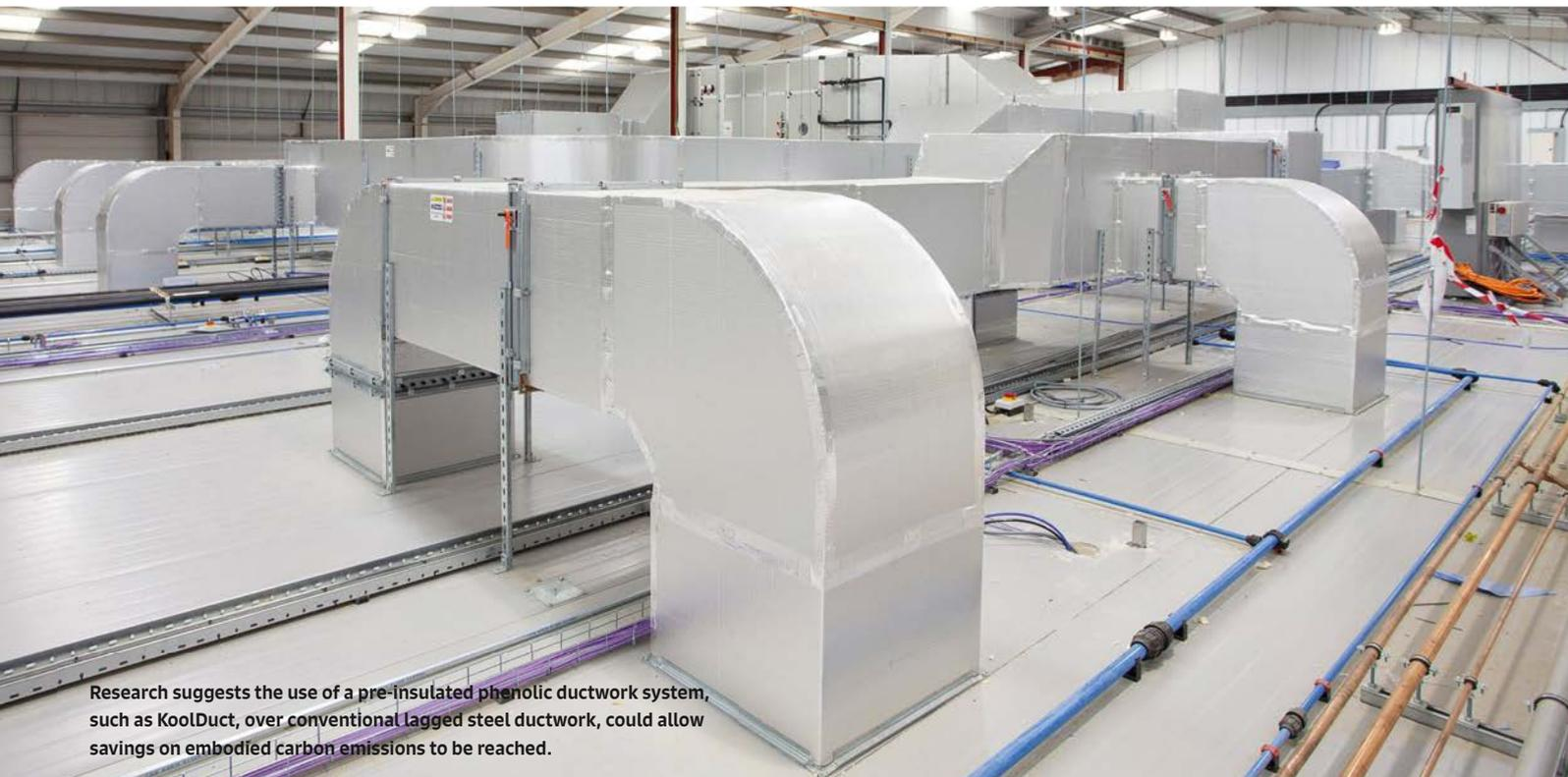
Research suggests the use of a pre-insulated phenolic ductwork system, such as KoolDuct, over conventional lagged steel ductwork, could allow savings on embodied carbon emissions to be reached.
