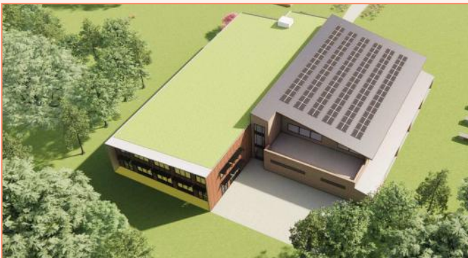
The Eco Center building is being designed to meet “passive house” building standards, with an aim of being the “greenest” building in Buffalo. These concept renderings of the building depict a green, living roof, and a rooftop solar array. Rendering by eco_logic STUDIO, architecture & engineering, PLLC.
