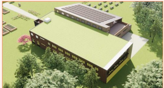
The Eco Center building is being designed to meet “passive house” building standards, with an aim of being the “greenest” building in Buffalo. These concept renderings of the building depict a green, living roof, and a rooftop solar array. Rendering by eco_logic STUDIO, architecture & engineering, PLLC.
