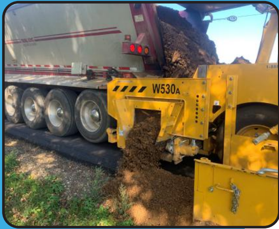
Placing shoulder gravel on XY Avenue
