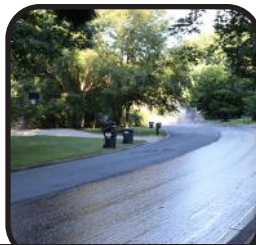
Chip/fog sealing on Rollridge Avenue
