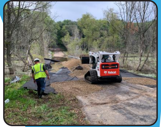
Aggregate lift on 8th Street bridge
