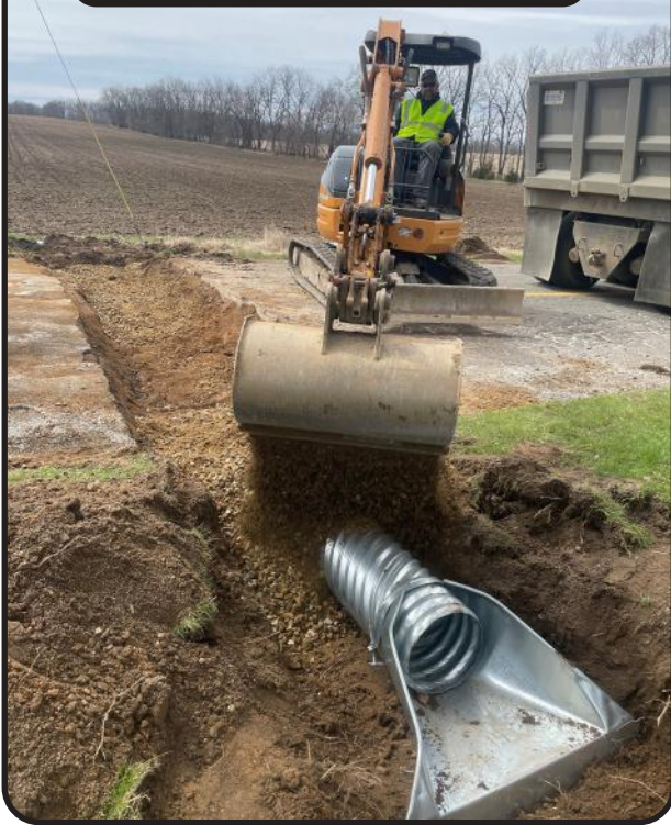
Cross culvert installation on V Avenue
