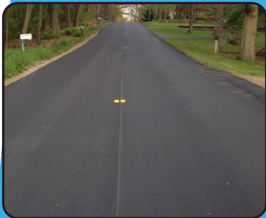
HMA paving on JK Avenue
