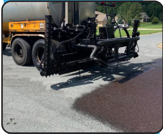
Fog seal in Oshtemo Township
