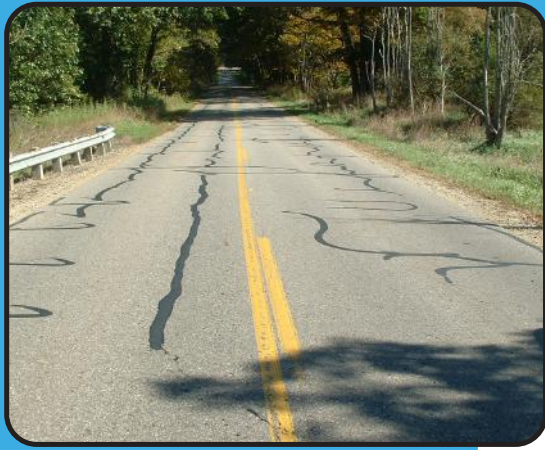
Crack seal on O Avenue
