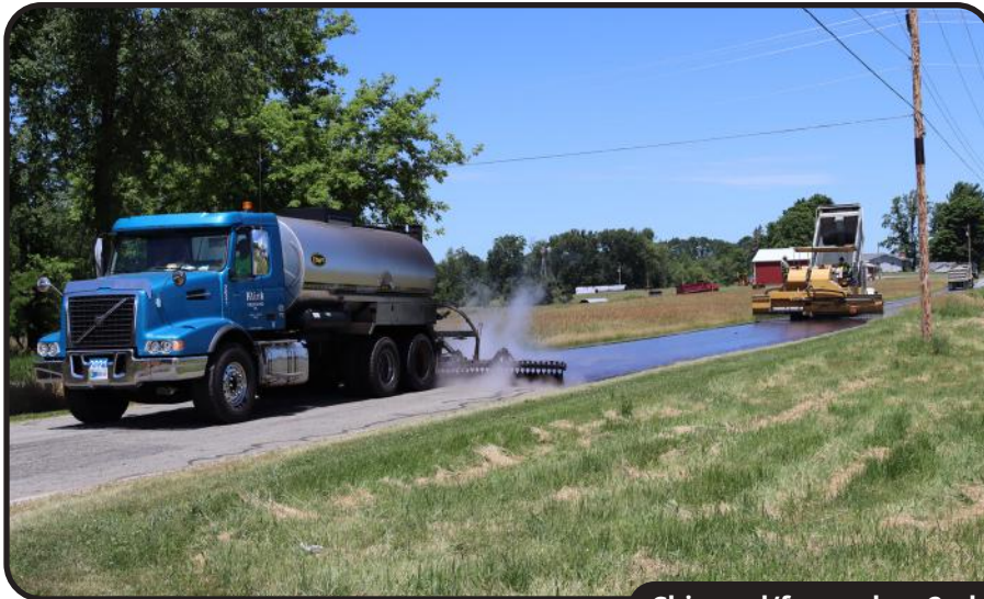
Chip seal/fog seal on 2nd Avenue
