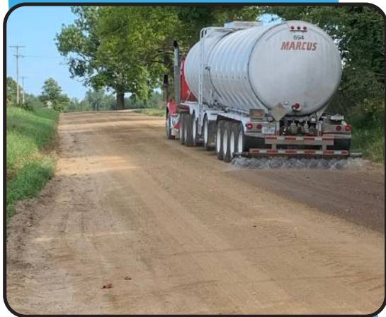
Applying dust control on 40th Street
