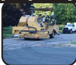
Chip/fog sealing on Rollridge Avenue
