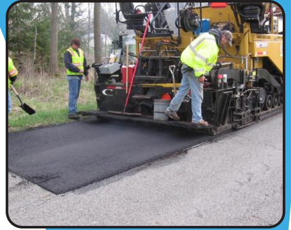
HMA wedge on V Avenue
