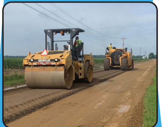
Pulverizing XY Avenue
