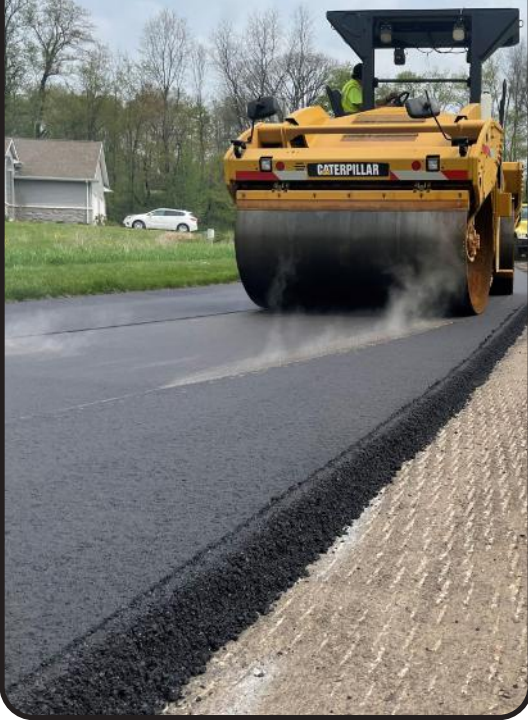
Paving on Old Savannah Drive
