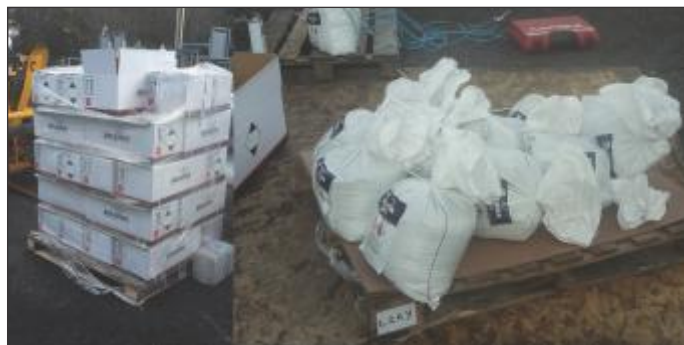
4,500 kg (9920.8 lbs) of Belzona 4131 (Magma-Screed).
