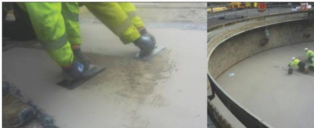
Belzona 4131 (Magma-Screed) applied using metal floats.
