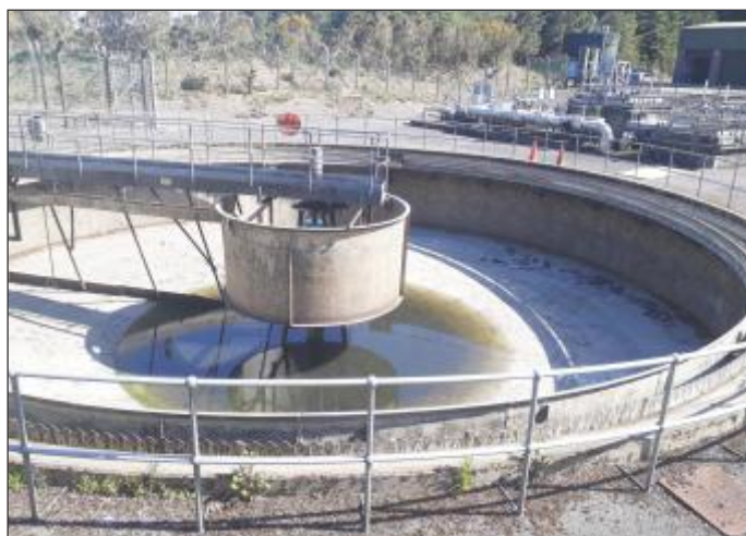
Tank drained one year on and found to be in excellent condition.
