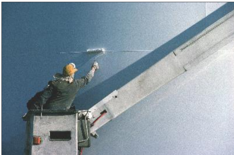
Paints that comply with standards such as those with low VOC emissions, high durability, and reflective properties are preferred for certified green buildings.
