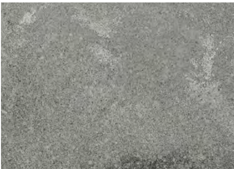
Metro Concrete R4
