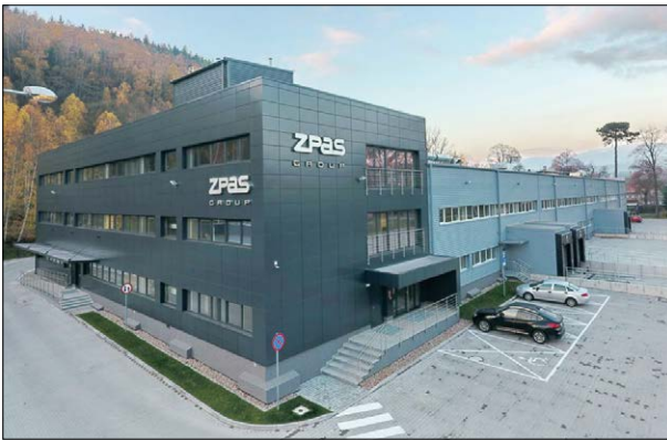
Nowa Ruda, Piłsudskiego Street Manufacturing plant – electrical assembly
