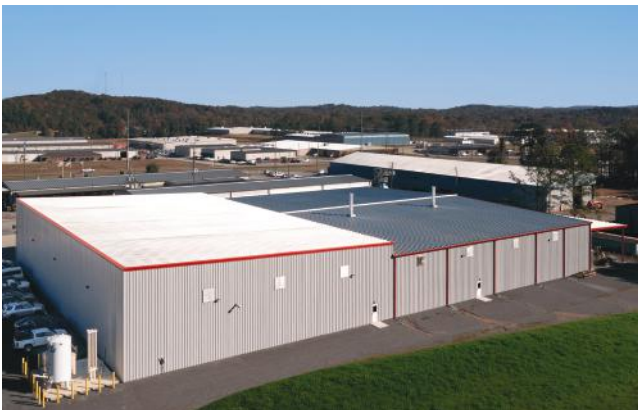
Douglas Manufacturing Pell City, AL BUILDER: Goodgame Company, Inc. | GC: Goodgame Company, Inc. ARCHITECT: Goodgame Company, Inc. Design Build Team
