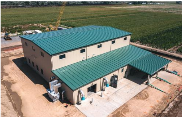
Johnstown Wastewater Treatment Plant MBR Building Johnstown, CO BUILDER: Baker Builders, LLC | GC: Moltz Construction ERECTOR: Baker Steel Erectors | ARCHITECT: Aqua Engineering
