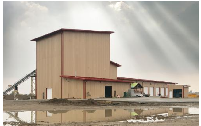
Croell Batch Plant Billings, MT BUILDER: Ainsworth-Benning Construction, Inc. | GC: Ainsworth-Benning Construction, Inc. ERECTOR: DDV, LLC
