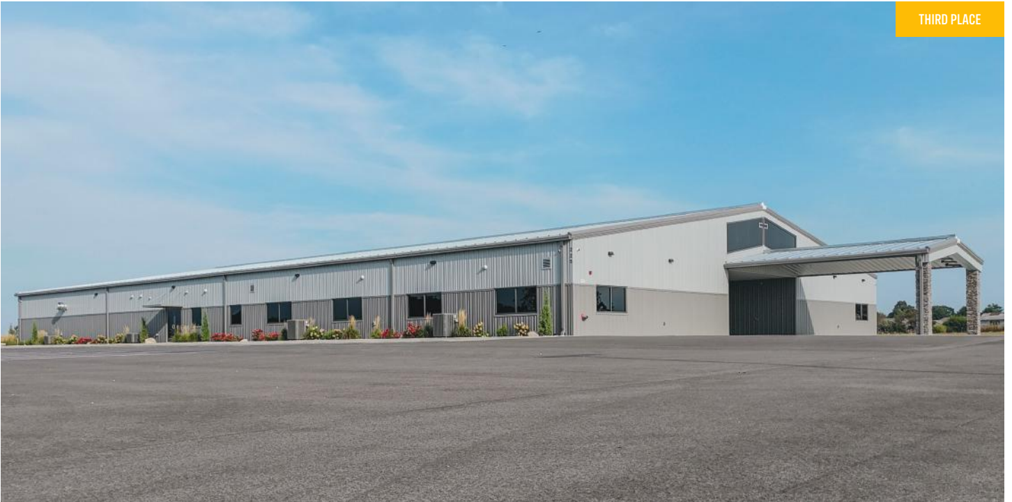
3 Summit Church Rogersville, MO | BUILDER: Williams Construction, Inc. | GC: Storee Construction | ERECTOR: Burk Erectors, Inc. | ARCHITECT: R.E. Werner
