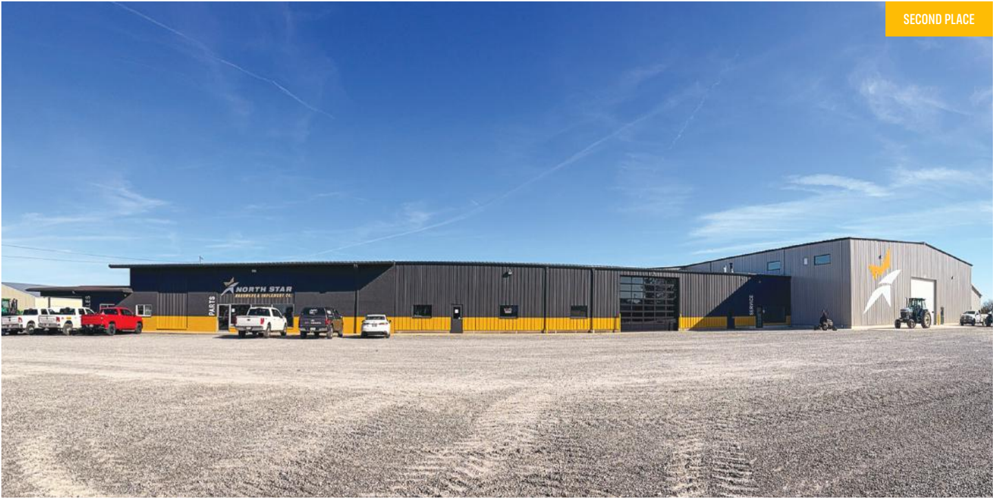
2 North Star Implement El Paso, IL | BUILDER: Bruns Building & Development | GC: Bruns Building & Development | ERECTOR: Bruns Building & Development | ARCHITECT: Bruns Building & Development
