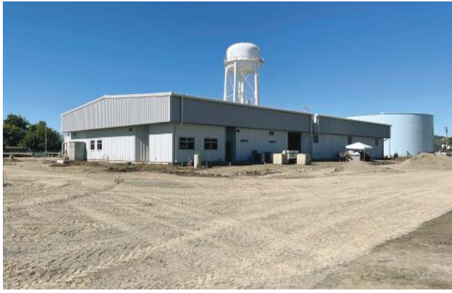
Dos Palos Water Treatment Plant Dos Palos, CA BUILDER: Gonzales Construction | GC: W.M. Lyles ERECTOR: All American Ironworks | ARCHITECT: AECOM
