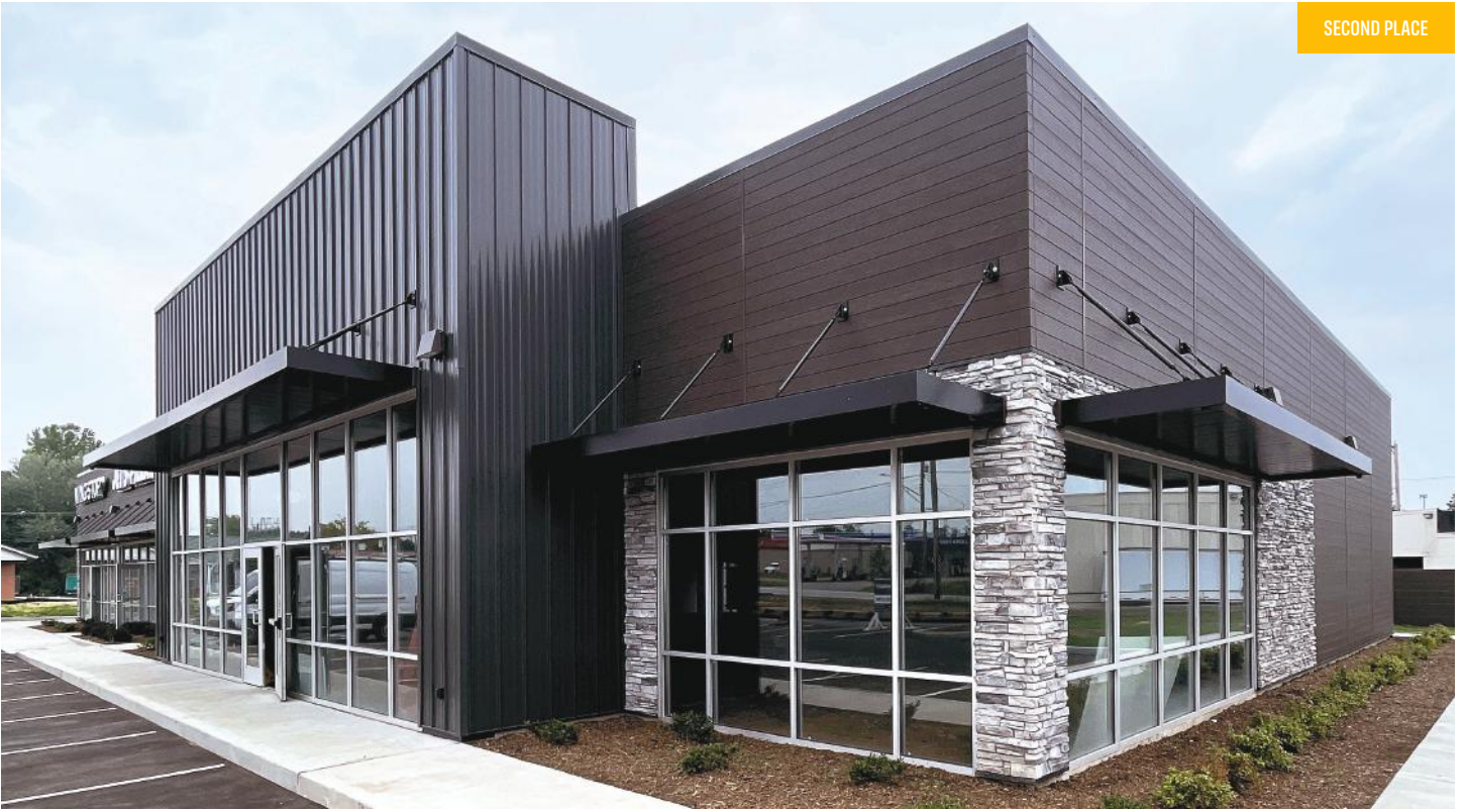
2 Westgate Place La Porte, IN | BUILDER: HGR Sales, Inc. | GC: HGR Group General Contracting | ERECTOR: HGR Group General Contracting | ARCHITECT: HGR Group
