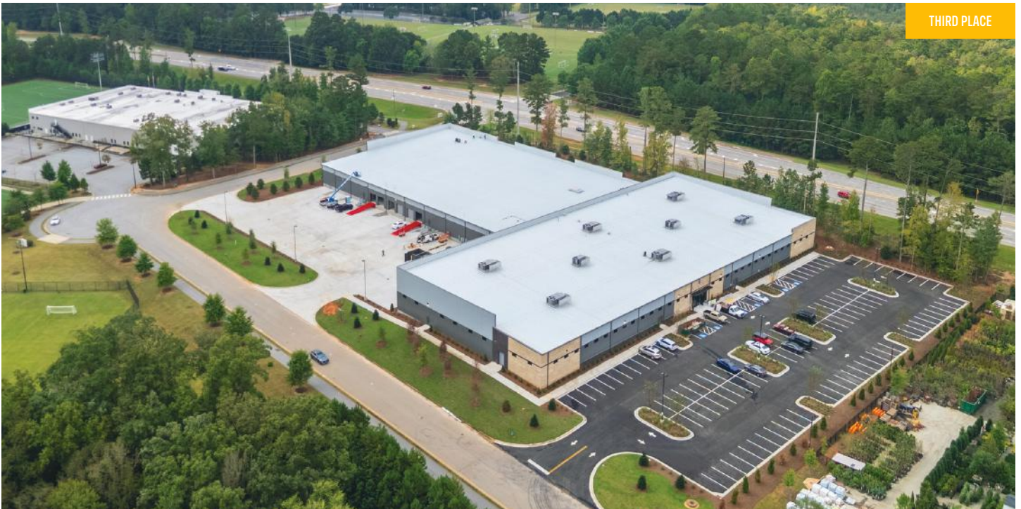
3 1001 Moba Peachtree City, GA | BUILDER: Southtree Commercial Construction, LLC
