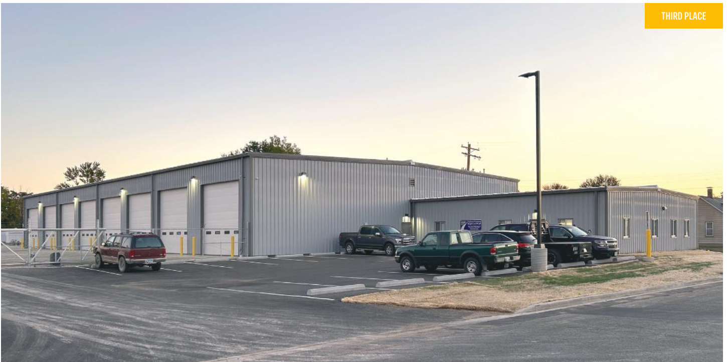
3 Fulton County Highway Department Maintenance Facility Canton, IL | BUILDER: Peoria Metro Construction | GC: Peoria Metro Construction | ERECTOR: Area Erectors, Inc. | ARCHITECT: Melotte, Morse, Leonatti, Parker, Ltd.
