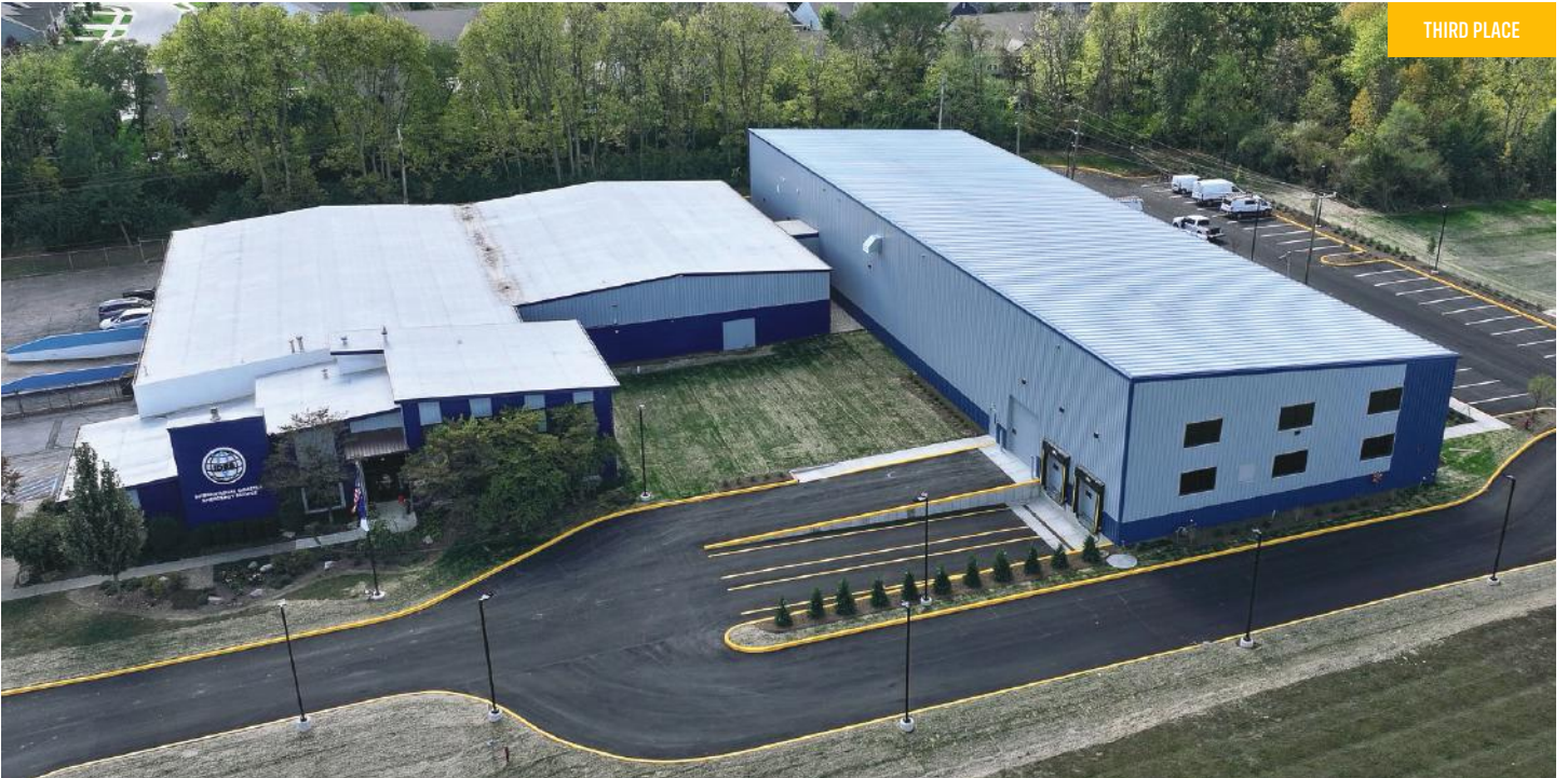
3 International Disaster Emergency Service Noblesville, IN | BUILDER: T&W Corporation | GC: T&W Corporation | ERECTOR: L&L Erectors | ARCHITECT: Site Architecture
