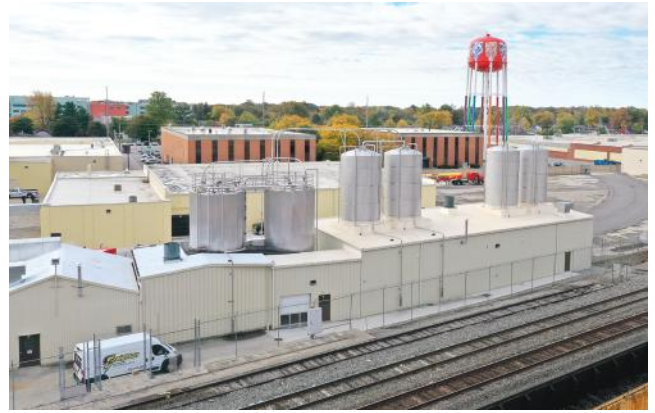
Spangler Candy Company - Sugar Shack Bryan, OH BUILDER: Thiel Construction Company, Inc. | GC: Thiel Construction Company, Inc. ERECTOR: Thiel Construction Company, Inc. | ARCHITECT: Bell Engineering
