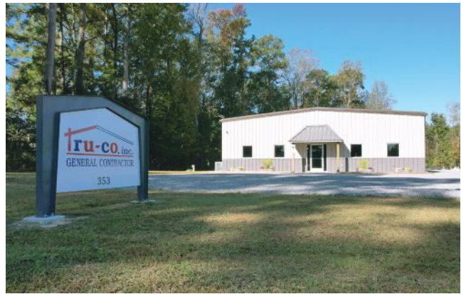
Tru-Co General Contractor, Inc. Office & Shop New Bern, NC BUILDER: Tru-Co General Contractor, Inc. | GC: Tru-Co General Contractor, Inc. ERECTOR: Edwards Erectors, LLC
