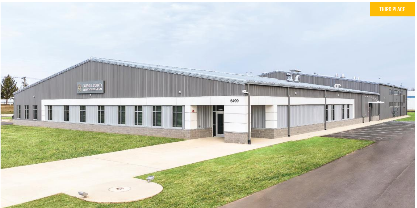
3 Carroll County Sheriff's Office & Jail Delphi, IN | BUILDER: Tri-Tech Construction Services, Inc.
