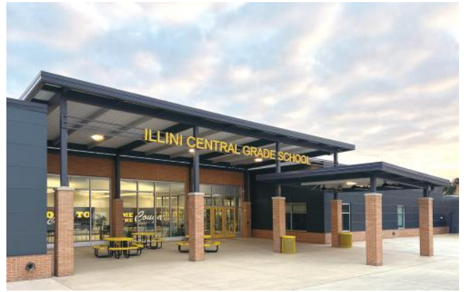
Illini Central Community Unit School District 189 Addition & Renovation Mason City, IL BUILDER: Peoria Metro Construction | GC: Peoria Metro Construction ERECTOR: Area Erectors, Inc. | ARCHITECT: PCM + Design Architects
