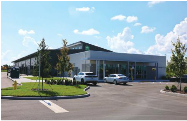
Manatee County Sheriff's Office Fleet Maintenance Building Palmetto, FL BUILDER: Mark Construction Company
