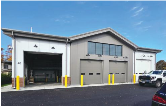
Dedham-Westwood Water District Storage Facility Dedham, MA BUILDER: International Ventures, LLC | GC: Seaver Construction, Corp ERECTOR: International Ventures, LLC | ARCHITECT: RGB Architects
