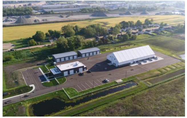
INDOT Mishawaka Unit and Salt Building South Bend, IN BUILDER: Hasse Construction Company, Inc. | GC: Hasse Construction Company, Inc. ERECTOR: SM Industries | ARCHITECT: Fosse & Associates
