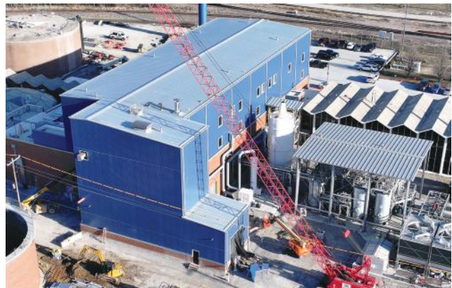
Blue River Wastewater Treatment Plant Kansas City, MO BUILDER: Cannon Building Systems | GC: Goodwin Brothers ERECTOR: Lane Ironworks | ARCHITECT: Black & Veatch
