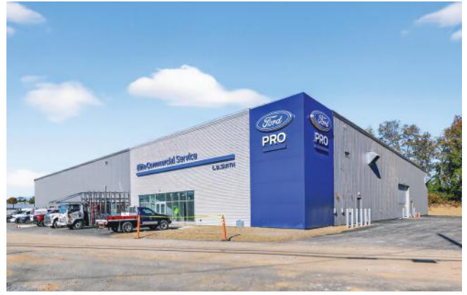
L.B. Smith Ford Elite Pro Commercial Service Center Camp Hill, PA BUILDER: E. H. Beiler Industrial Services, LLC | GC: JEM Group, LLC ERECTOR: E. H. Beiler Industrial Services, LLC | ARCHITECT: SGS Architects-Engineers, Inc.
