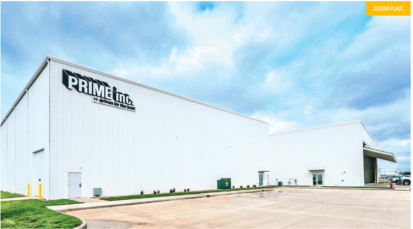
2 Killian - Prime Hangar Springfield, MO | BUILDER: Williams Construction, Inc. | GC: Killian Construction | ERECTOR: WilShar Steel, Inc. | ARCHITECT: Buxton Kubik Dodd Design Collective
