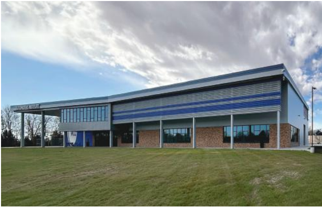
MCC Automotive Institute Lee's Summit, MO BUILDER: Weigel Construction, Inc. | GC: McCownGordon Construction ERECTOR: Weigel Construction, Inc. | ARCHITECT: DLR Group
