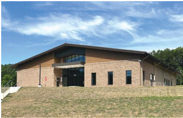
Woodbridge Seventh Day Adventist Church Manassas, VA BUILDER: Whitener & Jackson, Inc. | GC: Whitener & Jackson, Inc. ERECTOR: MTD Erectors, Inc. | ARCHITECT: Helbing Lipp Recny Architects
