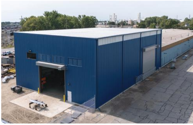
Vidimos Building Addition East Chicago, IN BUILDER: Hasse Construction Company, Inc. | GC: Hasse Construction Company, Inc. ERECTOR: SM Industries | ARCHITECT: CSK Architects
