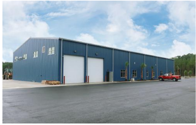
Cowboy USA Moncks Corner, SC BUILDER: Robbins Construction Group, LLC | GC: Robbins Construction Group, LLC ERECTOR: Cobb Industrial | ARCHITECT: Robert Johnson Architects
