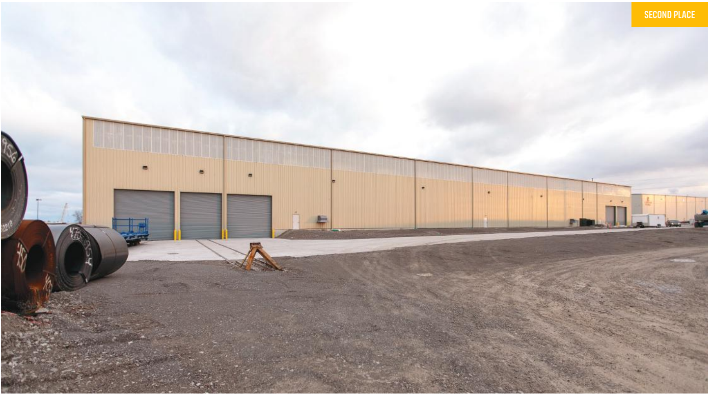
2 Feralloy Building Addition Portage, IN | BUILDER: Hasse Construction Company, Inc. | GC: Hasse Construction Company, Inc. | ERECTOR: Hampton Iron Works | ARCHITECT: Enspect, Inc.
