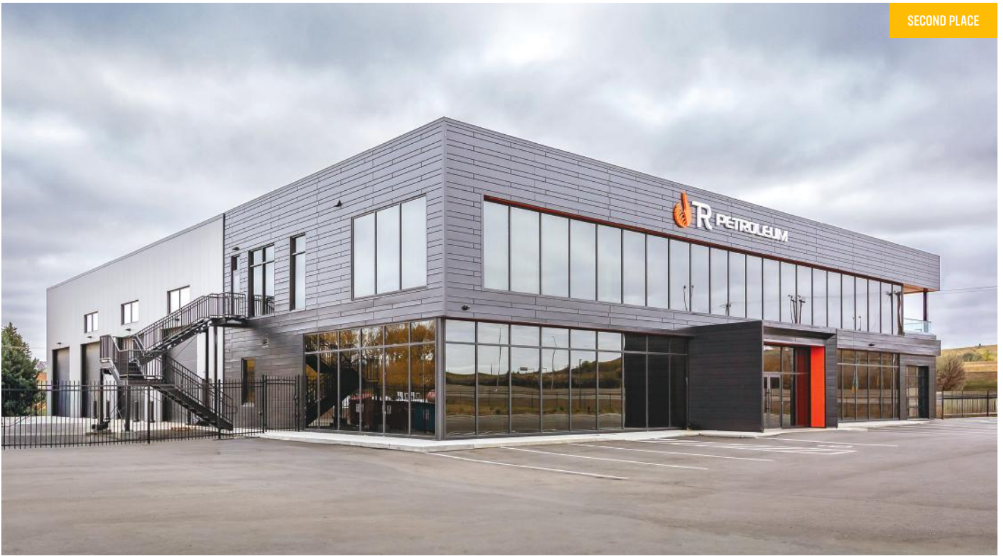
2 TR Petroleum Saskatoon, SK | BUILDER: Ledcor Design & Build Ltd. | GC: Ledcor Design & Build Ltd. | ERECTOR: Stratus Steel Erectors, Inc. | ARCHITECT: KSA Group Architecture
