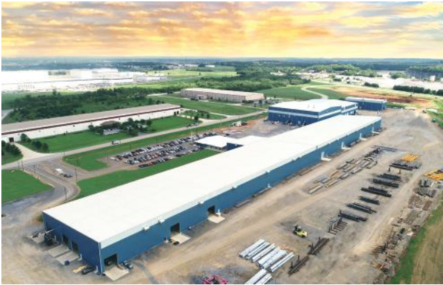
Nucor Towers & Structures Decatur, AL BUILDER: Fite Building Company, Inc. | GC: Fite Building Company, Inc. ERECTOR: Fite Building Company, Inc. | ARCHITECT: DIA
