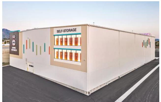
U-Haul U-Box Warehouse Murray, UT BUILDER: Petra, Inc. | GC: Petra, Inc. ERECTOR: Forge Building Company | ARCHITECT: Hillside Architecture
