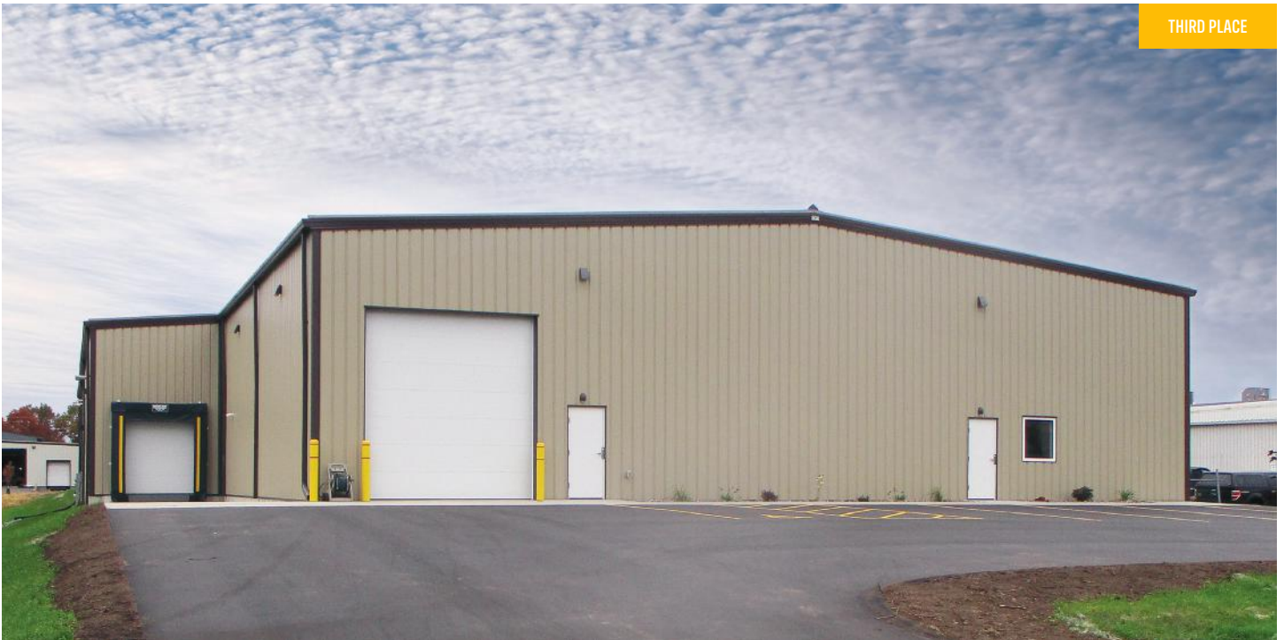
3 Louis Hogarth Warehouse Eau Claire, WI | BUILDER: Bauman Construction, LLC | GC: Bauman Construction, LLC | ERECTOR: Bauman Construction, LLC | ARCHITECT: Bauman Construction, LLC
