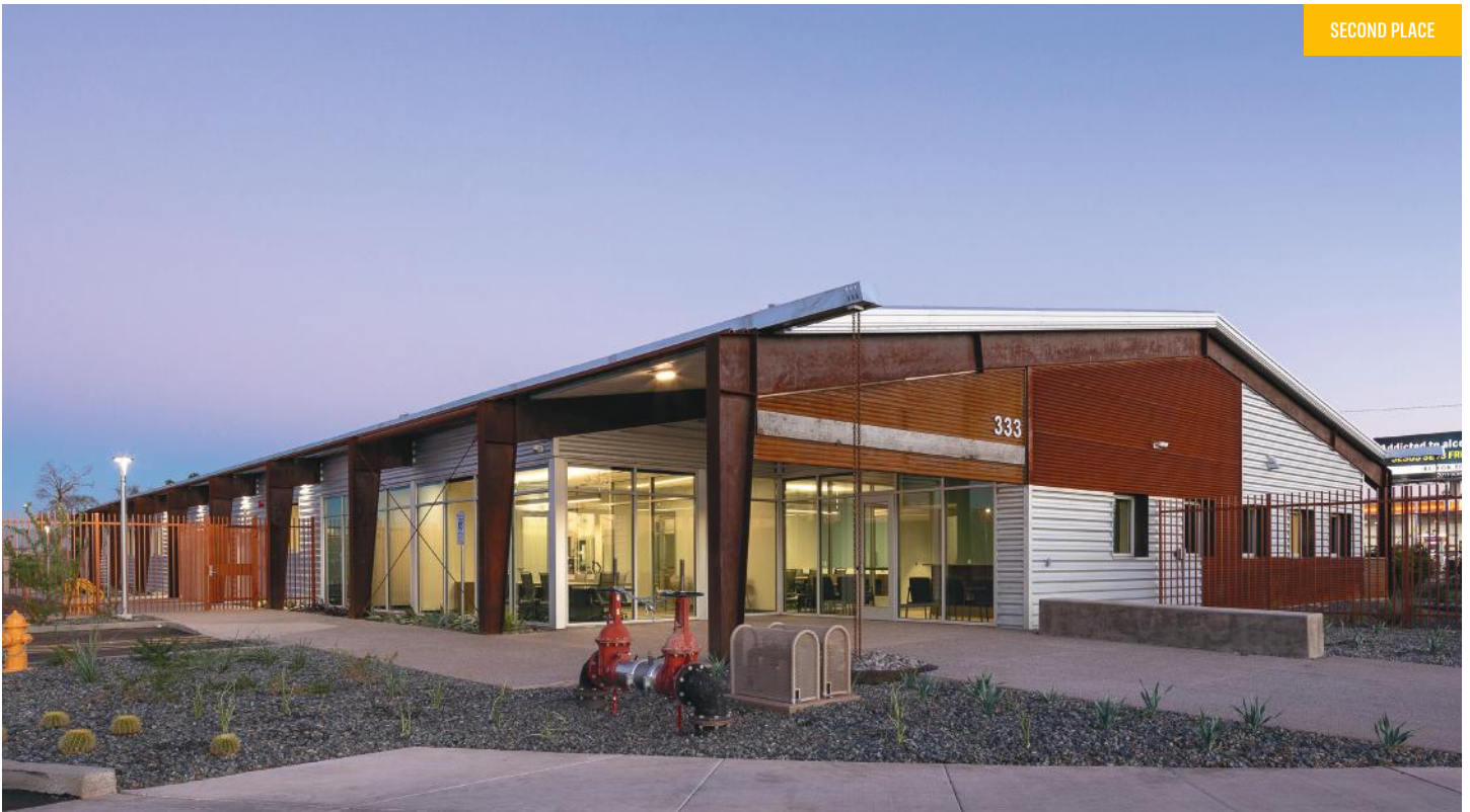
2 AHCCCS Transitional Shelter Phoenix, AZ | BUILDER: Colton Constructors, Inc. | GC: Colton Constructors, Inc. | ERECTOR: Eagle Erectors | ARCHITECT: LEA Architects, LLC
