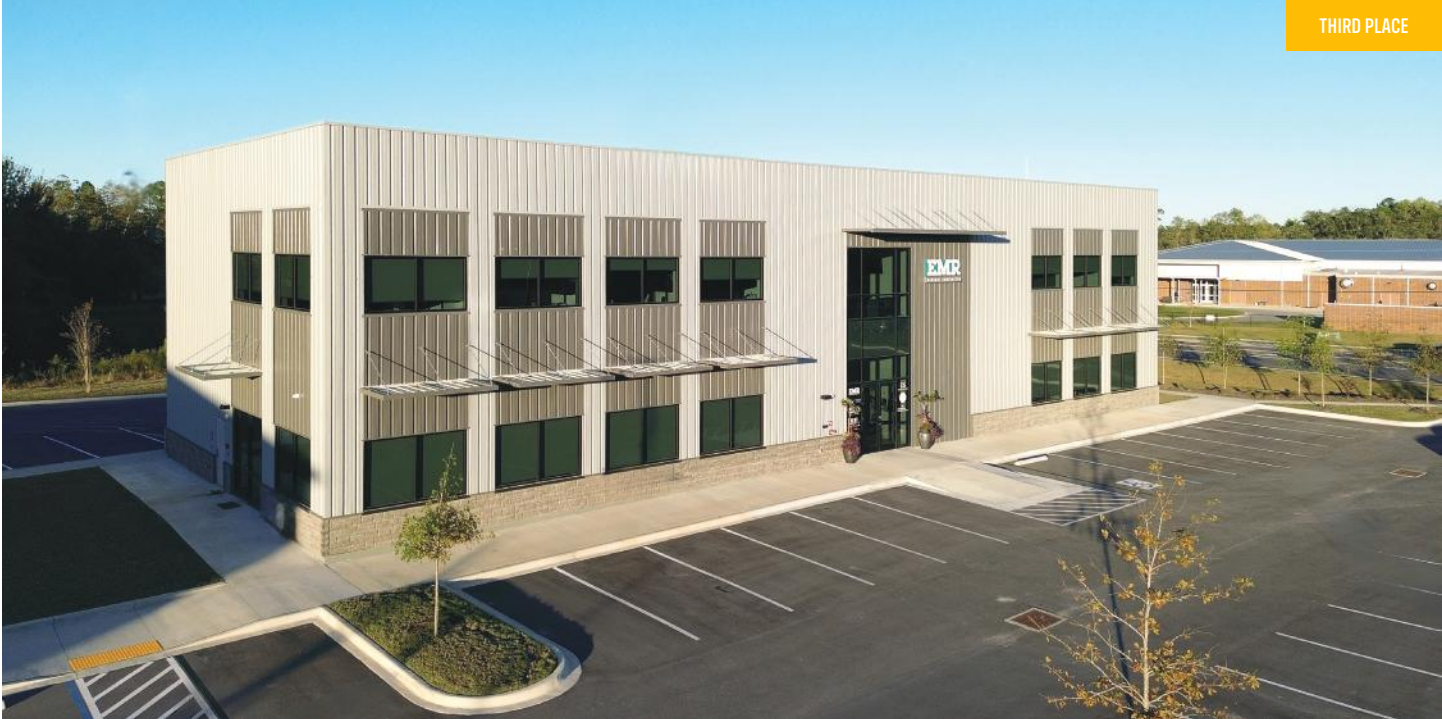
3 EMR Office Freeport, FL | BUILDER: EMR, Inc. | GC: EMR, Inc. | ERECTOR: Cheyenne Steel Erectors | ARCHITECT: The Jenkins Group
