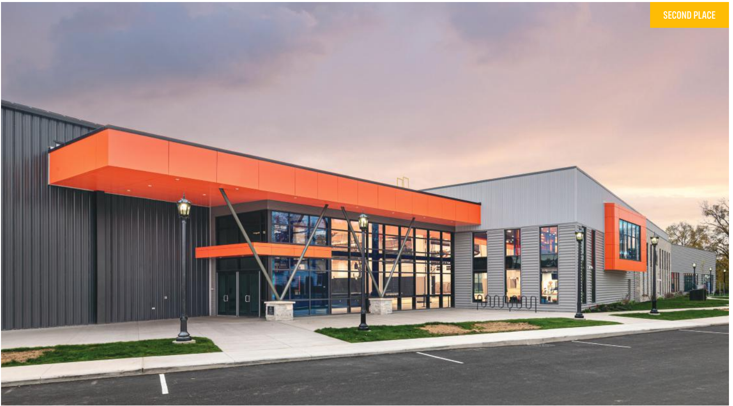
2 Frann's Fieldhouse Tiffin, OH | BUILDER: Marker Construction | GC: Marker Construction | ERECTOR: Steel Worx | ARCHITECT: Design Collaborative
