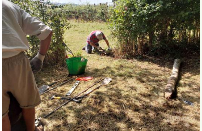
The gate posts on the Right of Way entrance to the wood had to be replaced - Photo: Judith Tranter
