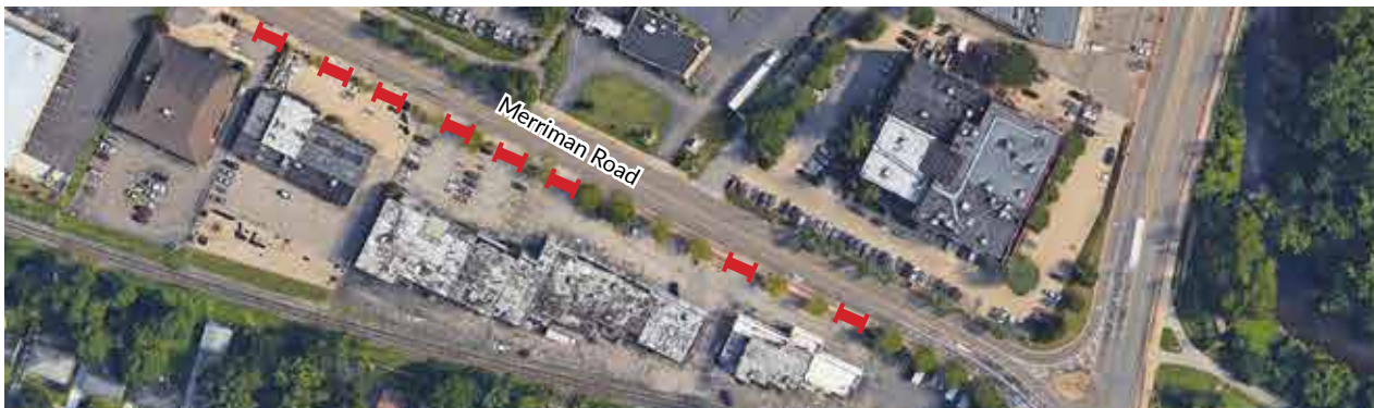
Figure 7.16 Conflict Zones Along Merriman Road for Pedestrians to Navigate. Source: Google Earth
