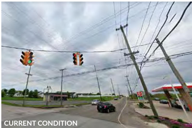
Figure 5.22 Maze of Power Lines Above Portage Trail Ext W / Northampton Road Intersection. Source: Google Street View
