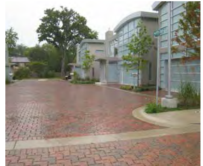
Figure 5.37 Permeable Paving. Copyright: Conservation Design Forum
