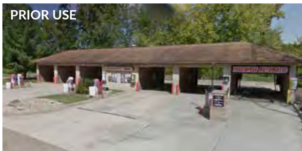
Figure 5.67 Car Wash Before Demolition. Source: Google Street View
