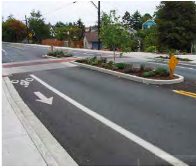
Figure 5.76 Pedestrian Refuge Example. Source: Wikimedia Commons, CC BY-SA 2.0
