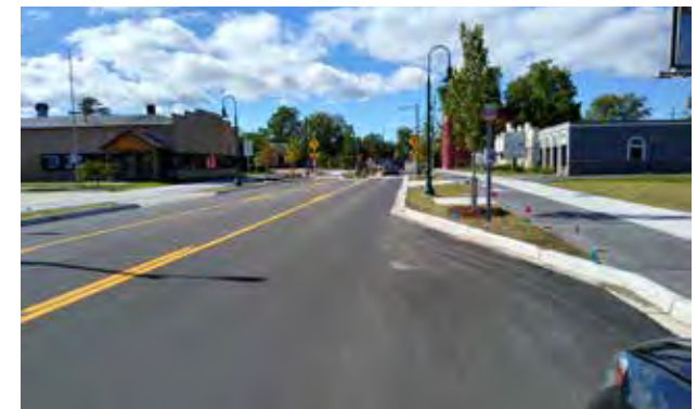
Figure 5.54 Successful Road Diet Implemented in Traverse City, MI, 23,000 ADT. Source: Farr Associates
