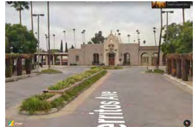
Figure 5.61 Glendale Station, CV Terminal Vista. Source: Google Street View
