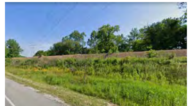
Above grade main sewer on Merriman Road
