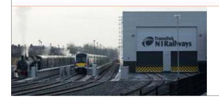
The works included the construction of a new train care maintenance facility on Translink's existing site in Adelaide, Belfast. The project comprised of a new train maintenance building, accommodation buildings and offices, refurbishment of an existing operations building and, infrastructure works including new HV distribution system, new train wash facility, fuelling apron and oil storage facilities.
