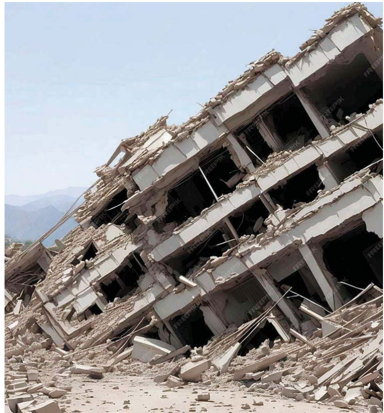
A building destroyed by a major earthquake. Photo: Supplied.
