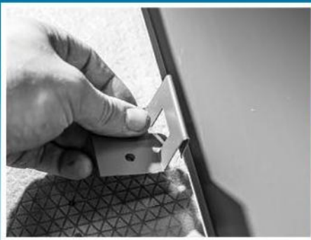
Attach the hidden clip to panel.
