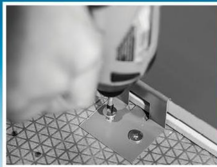
Fasten the hidden clip with pancake screws.
