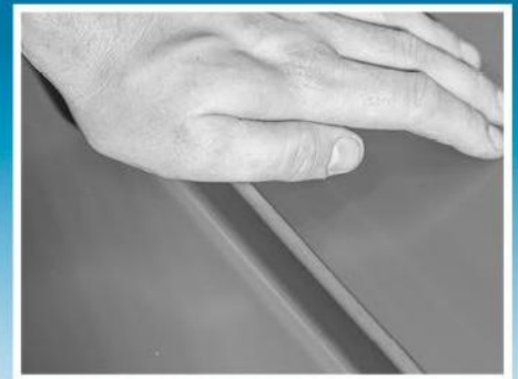
Snap the next panel in place.
