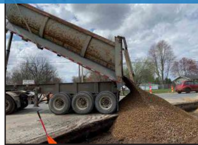
U Avenue chip seal/fog seal, and left-turn lane corrections
