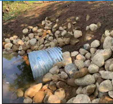
Culvert installations on CD Avenue
