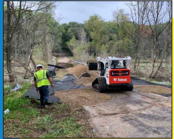
Aggregate lift on 8th Street bridge
