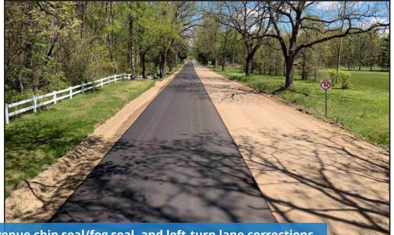
U Avenue chip seal/fog seal, and left-turn lane corrections
