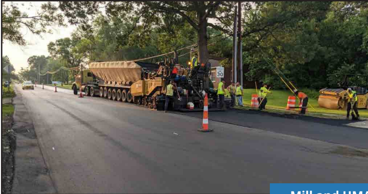
Mill and HMA overlay on G Avenue
