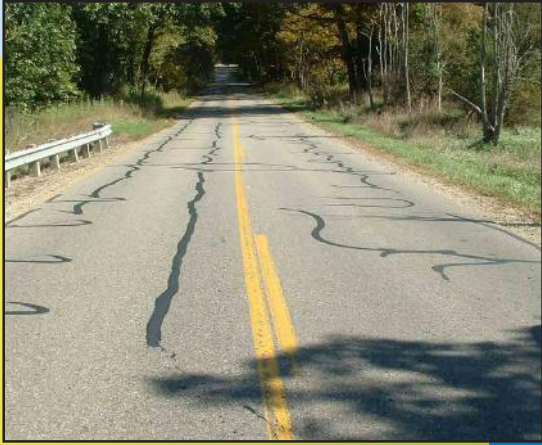
Crack seal on O Avenue
