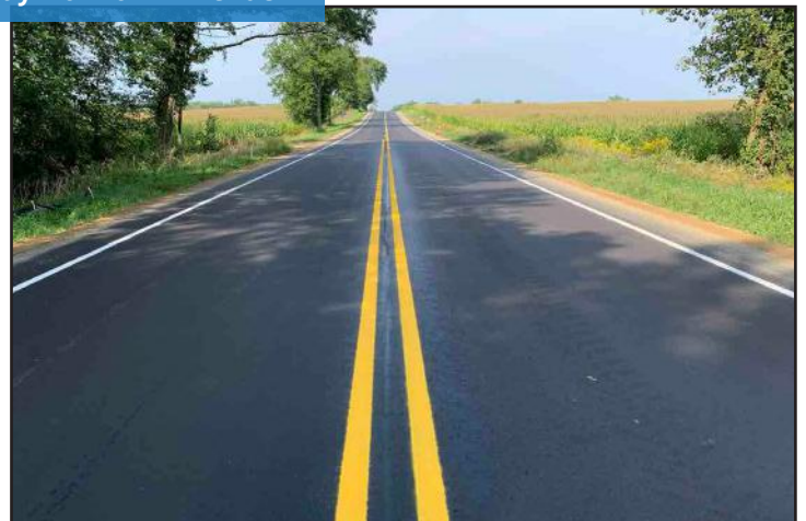
Mill and HMA Overlay work on R Avenue
