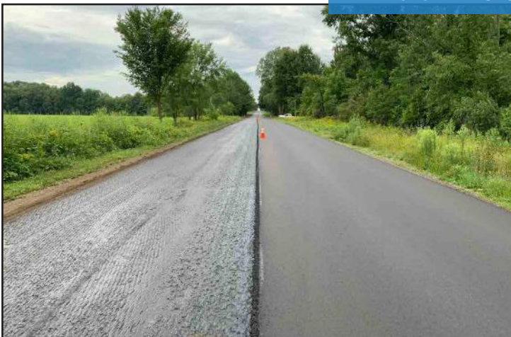
Mill and HMA Overlay work on R Avenue
