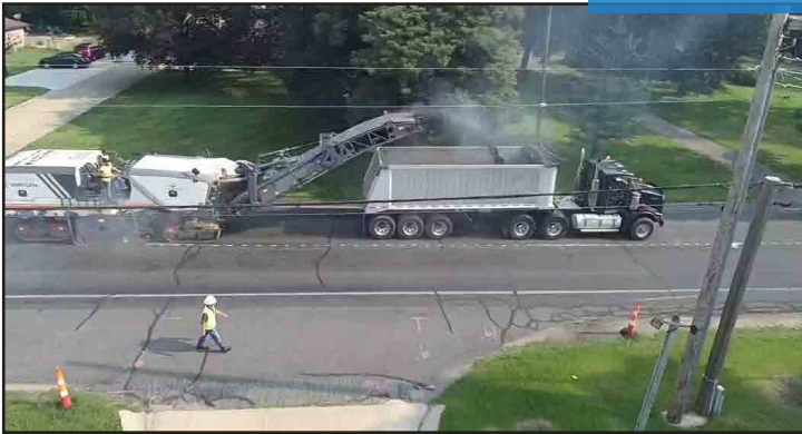
Mill and HMA overlay on G Avenue
