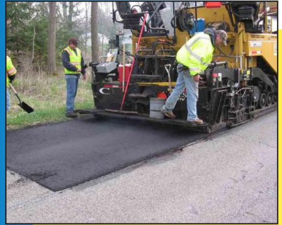
HMA wedge on V Avenue
