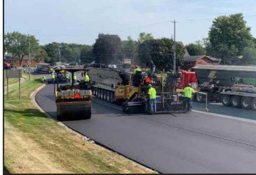
Nichols Road project - milling, HMA paving, drainage, and signal work
