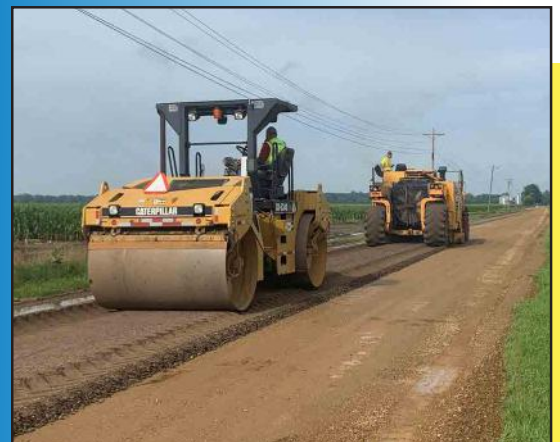
Pulverizing XY Avenue
