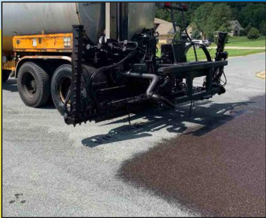
Fog seal in Oshtemo Township
