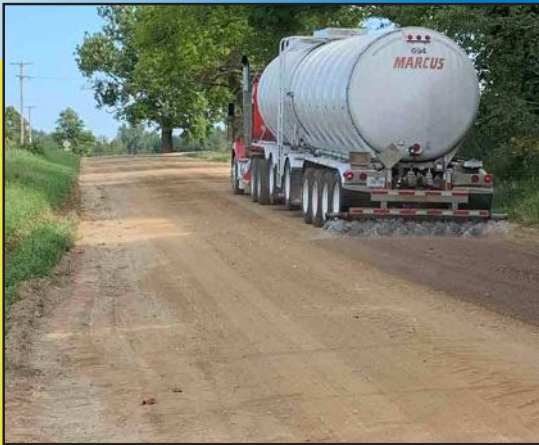
Applying dust control on 40th Street
