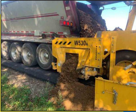
Placing shoulder gravel on XY Avenue
