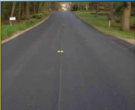
HMA Paving on JK Avenue
