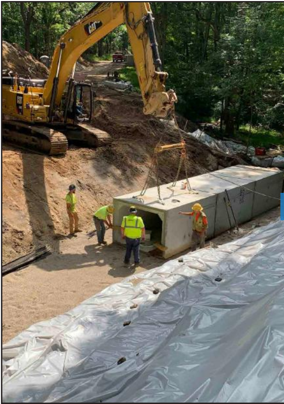
Culvert installations on CD Avenue
