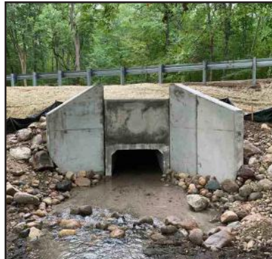
Culvert installations on CD Avenue
