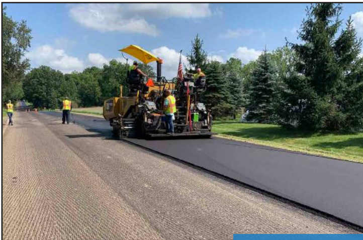
Mill and HMA Overlay work on R Avenue
