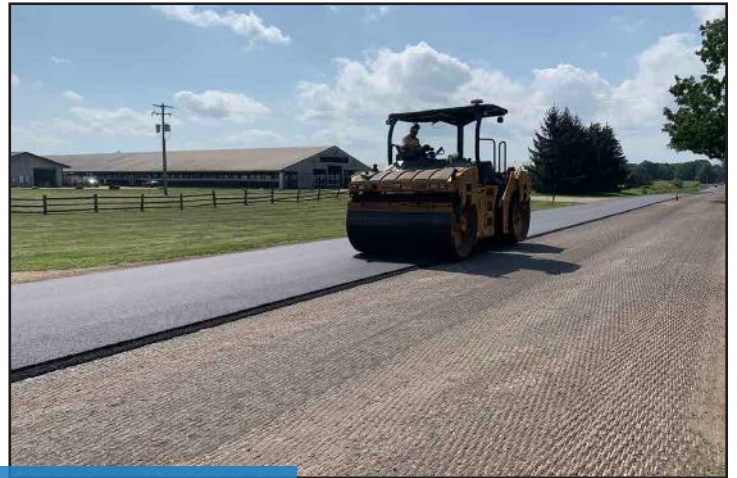
Mill and HMA Overlay work on R Avenue
