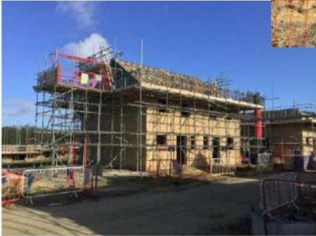
Affordable homes being built in Cottenham
