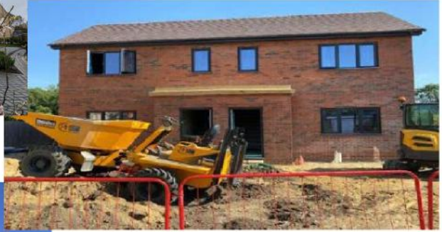
Affordable homes being built in Orwell
