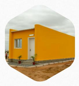
Power2Build used the Dfab material solution, a ground-breaking concrete mix developed by COBOD and CEMEX, achieving cost savings of 90%. This was because 99% of the material was sourced locally, and only 1% was provided by COBOD. Power2Build was the first to print with this solution, pioneering the concrete revolution of 3DCP.
