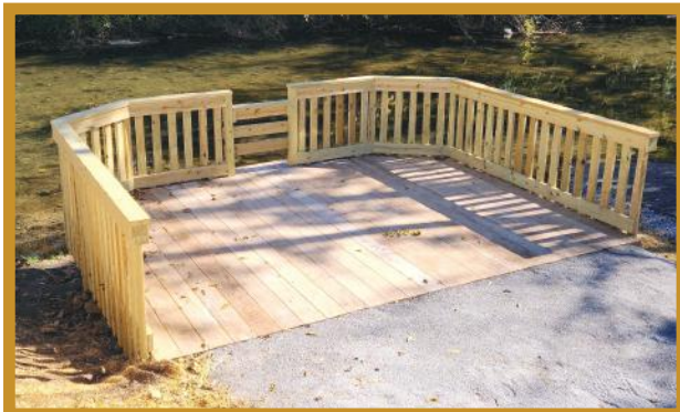
Fishing Dock and Canoe/Kayak Launch constructed in 2025. Funding provided by Pennsylvania Fish and Boat Commission through the Boating Facilities Grant program.
