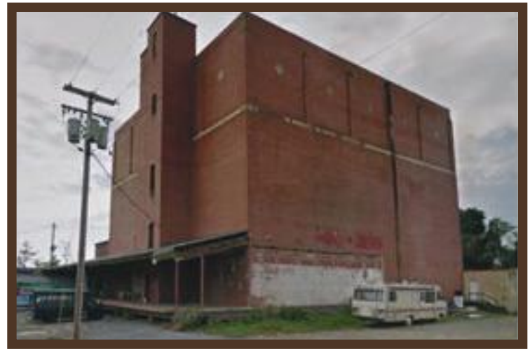
Former Building Demolished.
