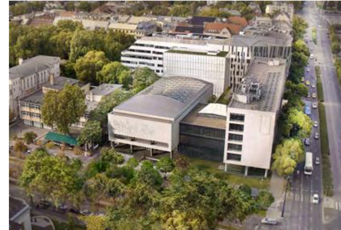
LIGET CENTER CLASSIC, AUDITORIUM AND VITRUM OFFICE BUILDINGS
