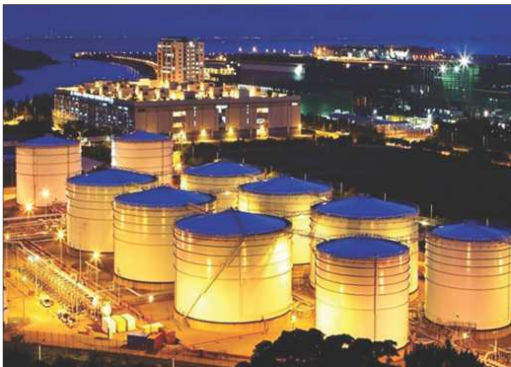
Considering that highly vulnerable materials such as petrochemicals or chemical gases are stored in the tanks, improper coating can also bring about the contamination and dilution of these chemicals.
