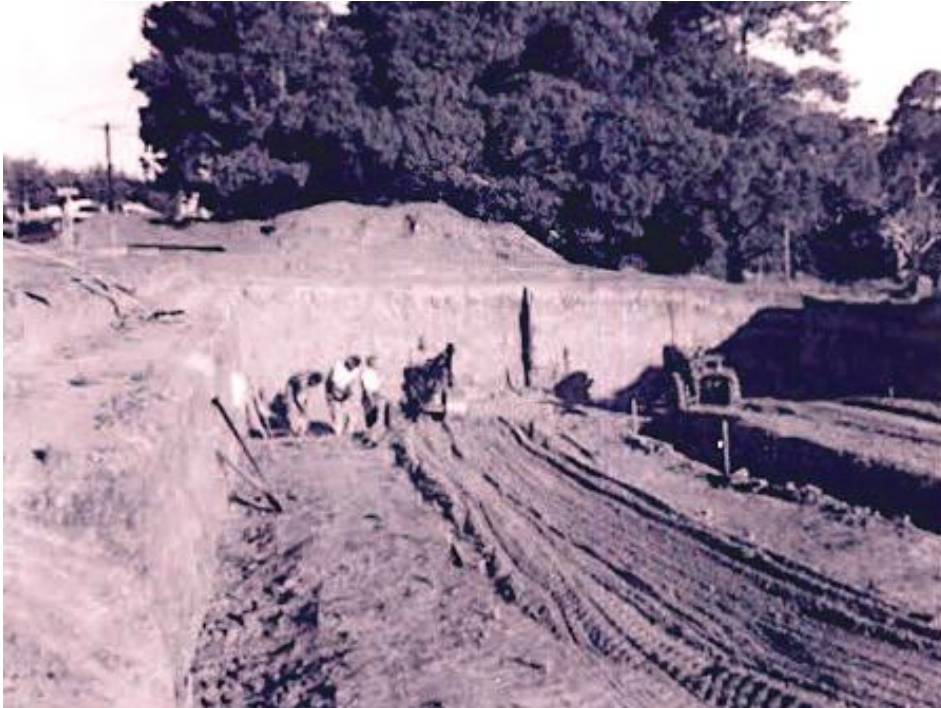
Construction of Swimming Pool, Winchelsea 1962
