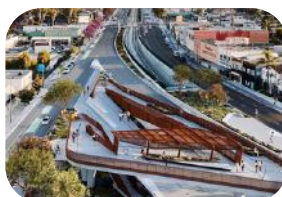
Council District 8 Marqueece Harris-Dawson Destination Crenshaw
