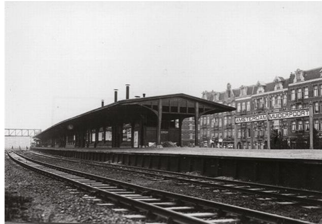
Houten eilandstation Muiderpoort I, 1910. [HUA]
