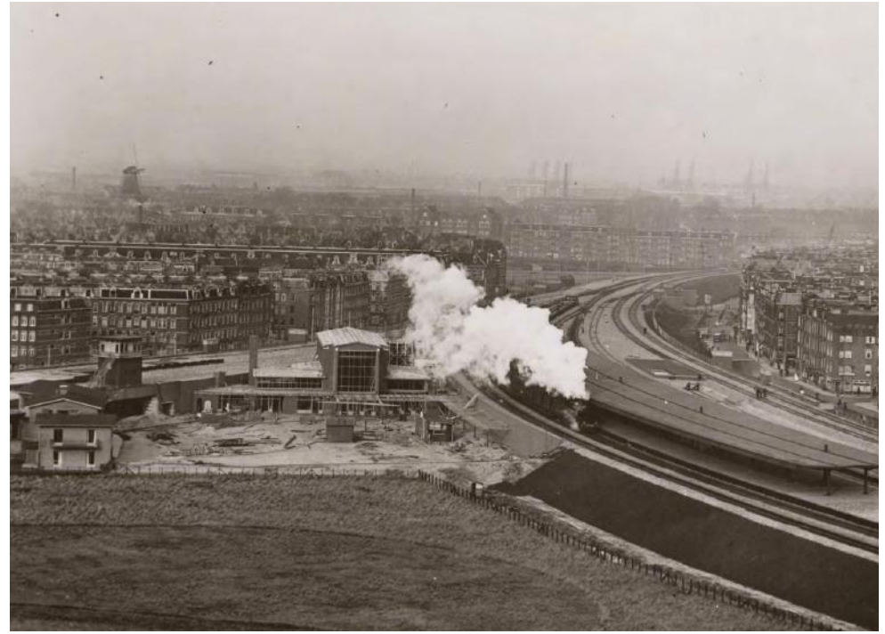
Station Muiderpoort in aanbouw, 1939. [SAA]
