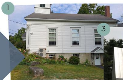
Picture 1 & 2 New Energy Efficient Heat Pump System Wayne ME
