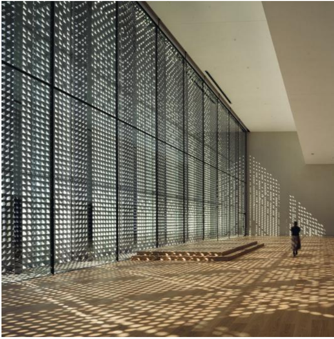
Left: The huge south wall stone screen and glazing to the upper-level social hall. Steel posts supporting the screen are rendered almost invisible by mirror-steel cladding.
