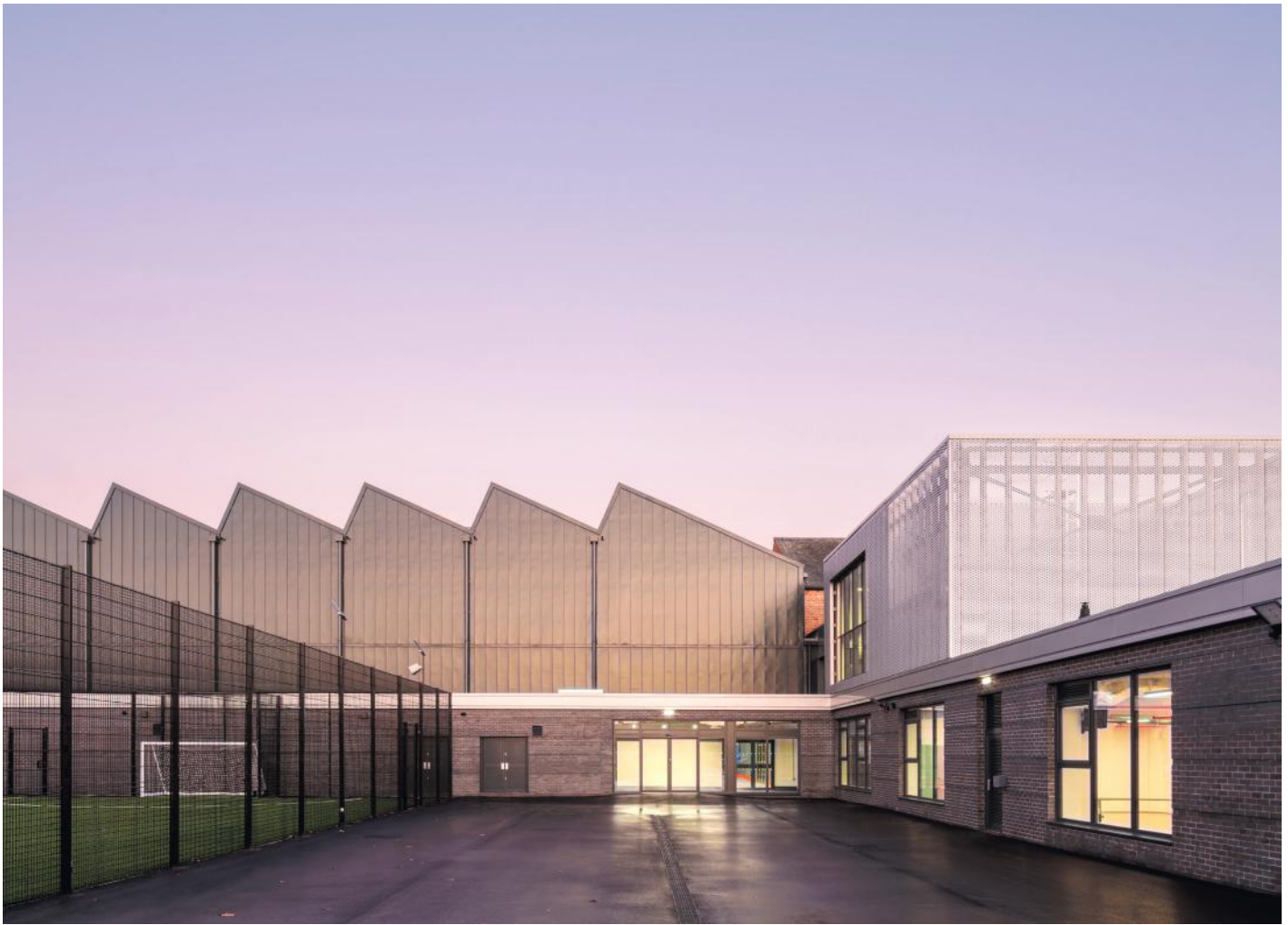
Above: New construction includes a climbing wall wrapped in expanded aluminium mesh.
