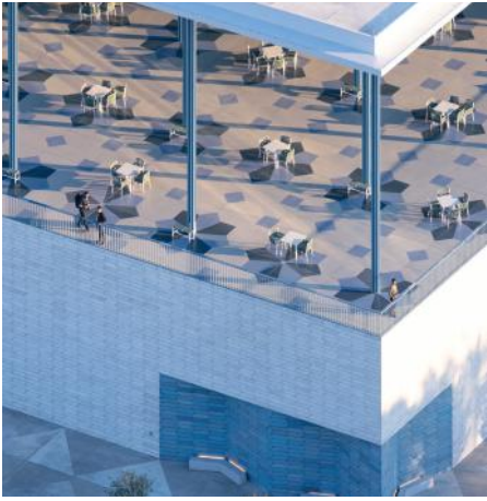
Above: Outer Prayer Hall corners both have garden seating alcoves, cast in the same blue-tinted UHPC that forms eivan soffits.
