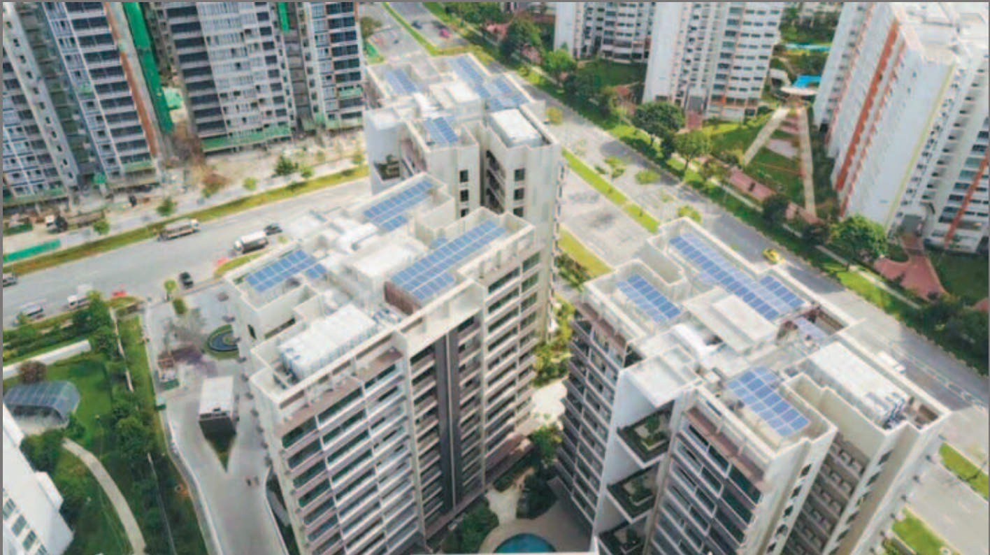
Residential Blocks with Photovoltaic Panels
