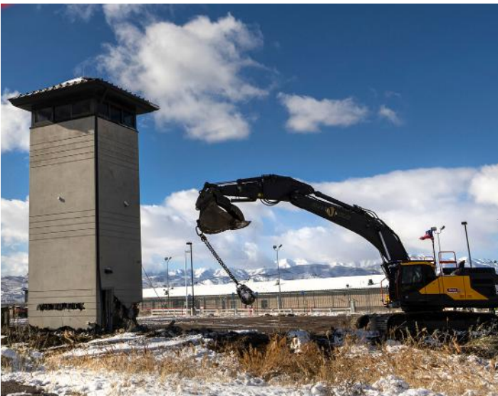
Figure 12: Total demolition of the Utah State Prison.
