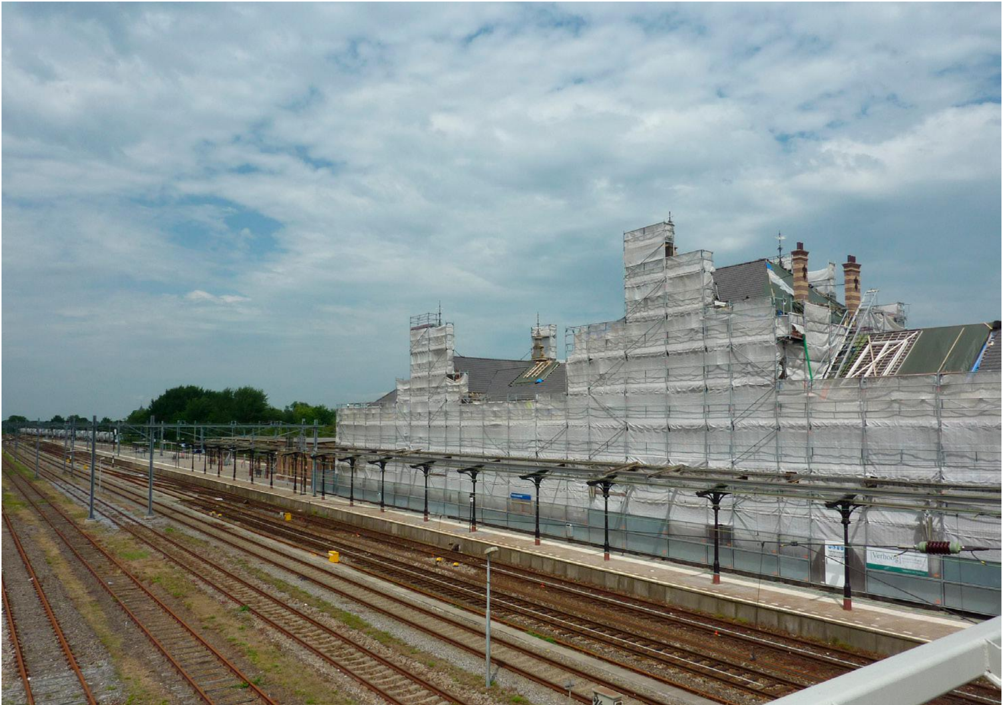
Station Geldermalsen in restauratie.
