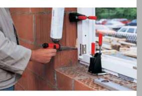
■ Permits rapid, precise straightening and fixing of window frames
