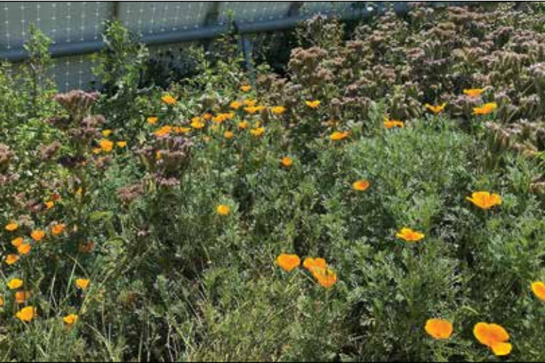
A mixture of wildflower species attracts pollinators around and beneath solar panels at a UC Davis ecovoltaic project.
