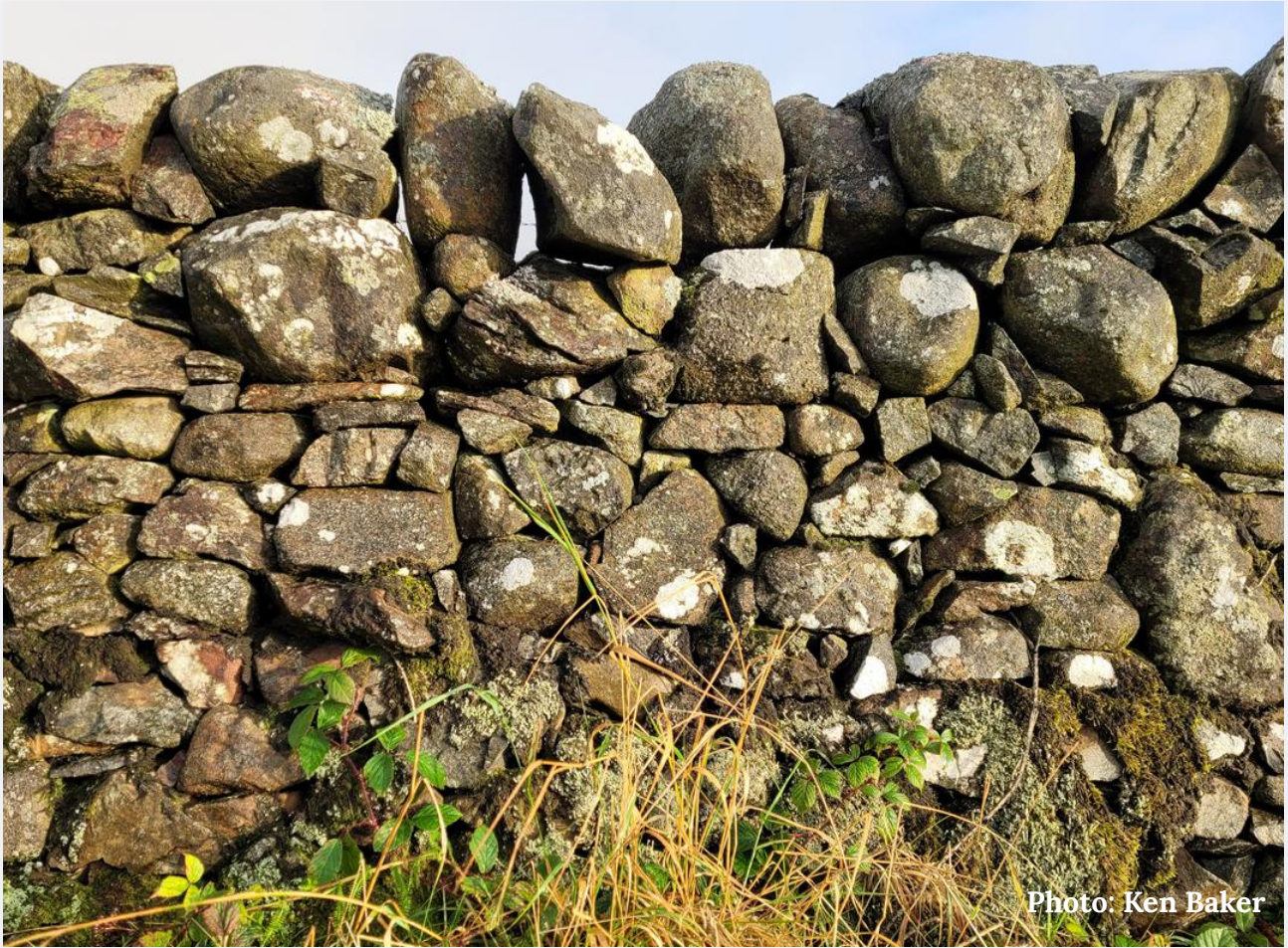
A section of a collapsed dyke showing the importance, of 'ties' when building with this type of stone
