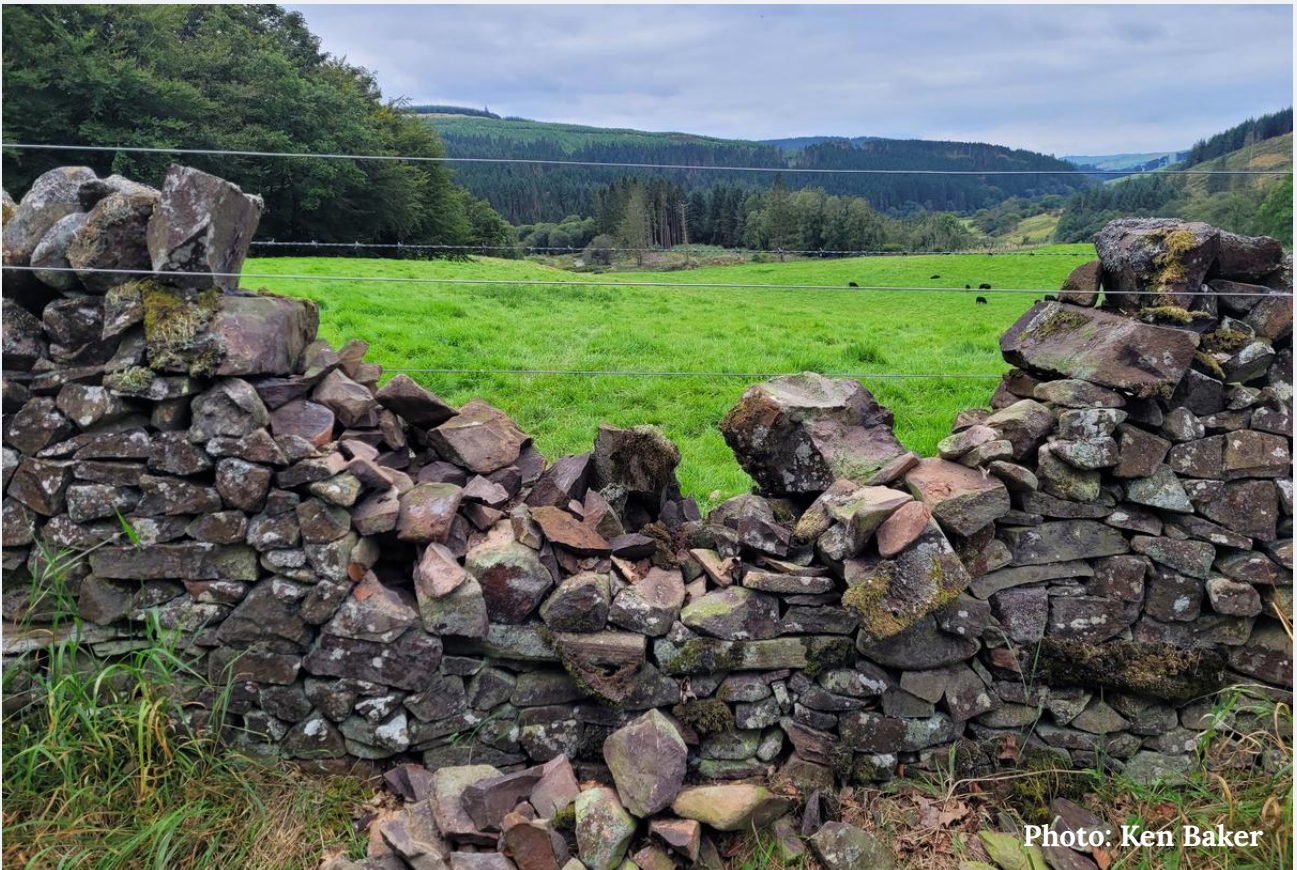
A section of a collapsed dyke showing the importance, of 'ties' when building with this type of stone
