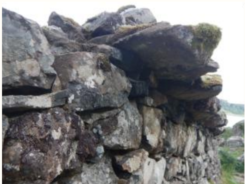
This photo, from the Isle of Sky, shows a wall with overhanging copestones. These overhangs were around 250 mm on both faces of the wall.
