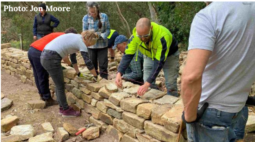
Carey Gully Sandstone being used in a dry stone walling workshop in the Adelaide Hills, South Australia.
