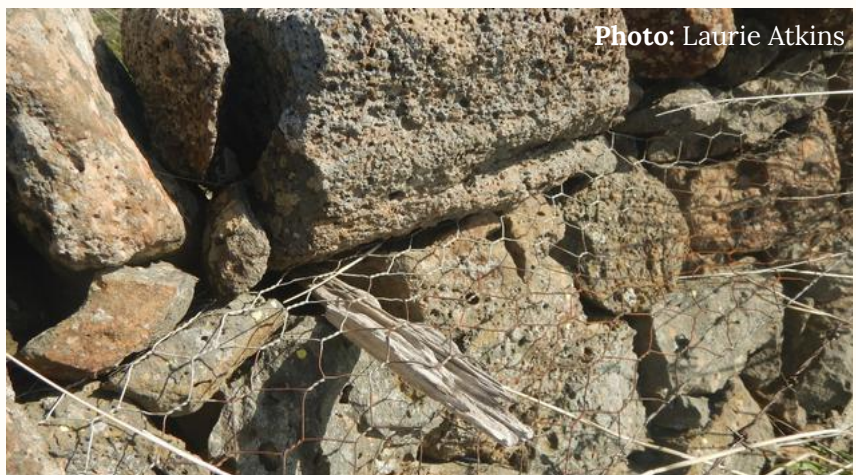
A wall at Bamganie (near Lethbridge), Victoria, shows a section of regulation, free standing double DSW with wire mesh placed under the copestones and held horizontally on both sides by the remnants of a narrow timber slat. A run of barbed wire was fixed to the margin of the mesh indicating the need for a defense against sheep.
