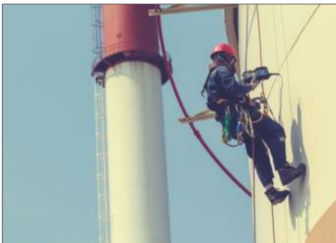
On-site inspection of a storage tank.
