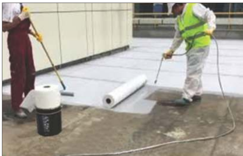
Waterproofing is the process of making a surface or structure resistant to water by applying a protective barrier, which prevents water from penetrating and causing damage.
