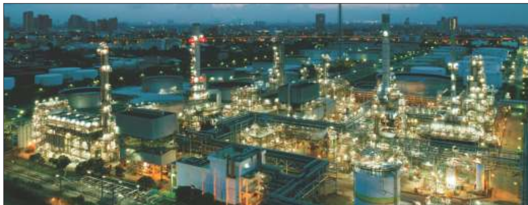
Given the cost of engineering, procurement and construction of process installations, the ultimate successful facility is one that remains in the intended service for as long as possible.
