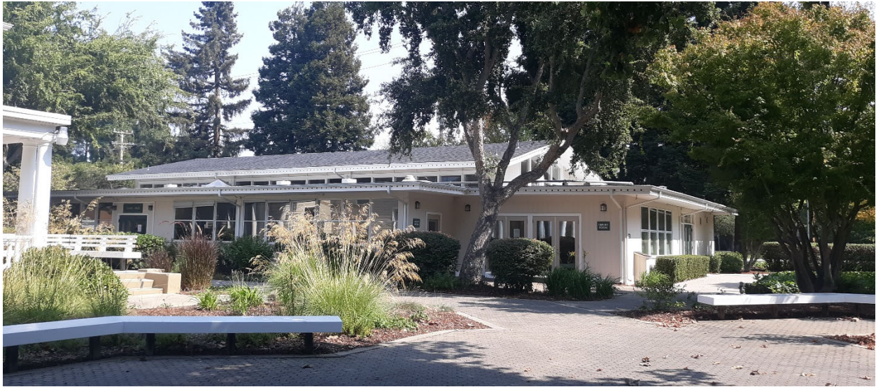
Figure 1: Trinity Hall has high potential for photovoltaics.
