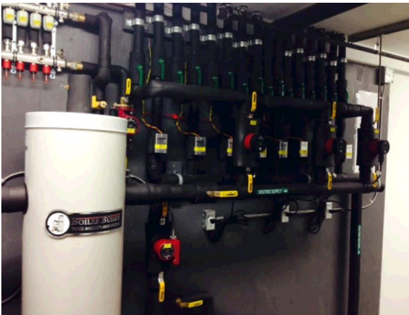
Figure 3: Example Hydronic System
