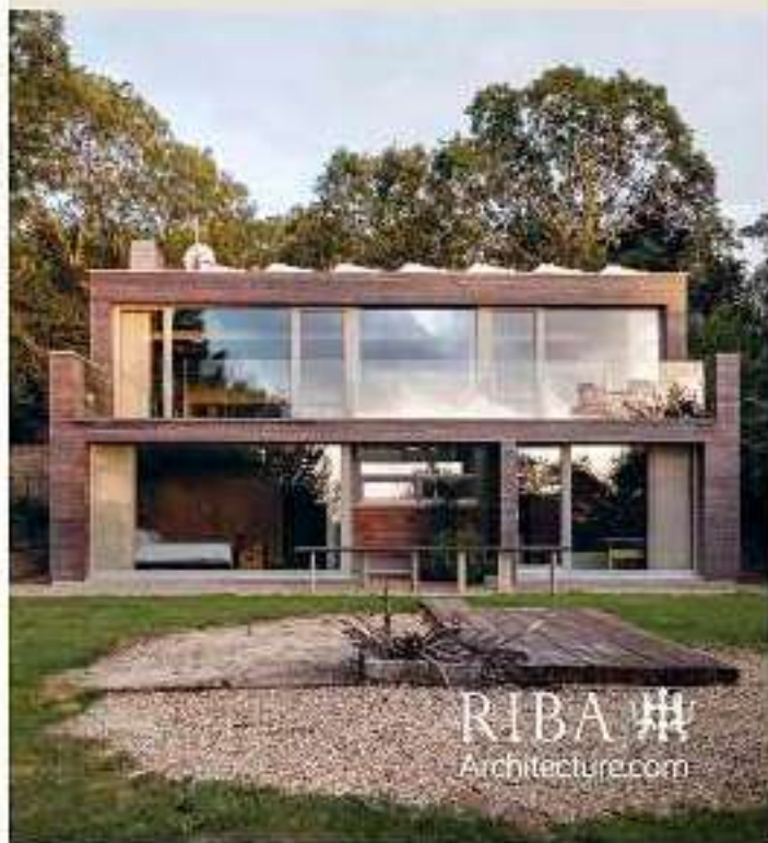
Heads, surrounds, sills, balcony mouldings are FoamStone®
