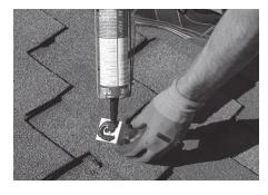
Apply sealent to the bottom of the Tamarack L-foot mount.
