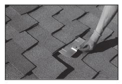
Slide flashing under the shingle course above the pilot hole. Position hole in flashing directly over the pilot hole. Use a pry bar to lift up shingles if necessary.
