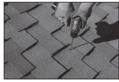
Drill a 7/32" pilot hole for the lag bolt. Drill through the roofing material and into the framing member.
