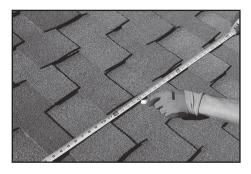
Locate roof attachment points directly over the center of the rafter and 1-1/2-inches below the shingle above the hole.
