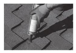
Apply a good quality flashing sealent in and around the pilot hole.
