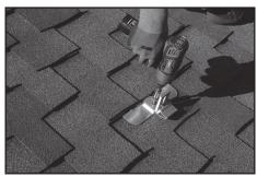
Insert the lag bolt through the sealing washer with the rubber side down and drive the bolt into the hole.
