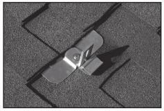
Tighten the lag bolt so the sealing washer is tight against the flashing.
