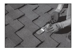
Place L-foot base under the hole in the flashing so that the hole in the L-foot lines up with the hole in the flashing, directly over the pilot hole.
