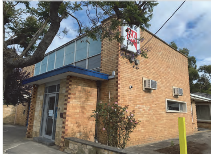
Bank SA, Yankalilla, on 10 December 2022, the day after final closing.
