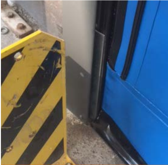
Heavy-duty zip system and FlexEdge bottom beam
