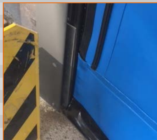
Guide rail with zip system and FlexEdge bottom bar
