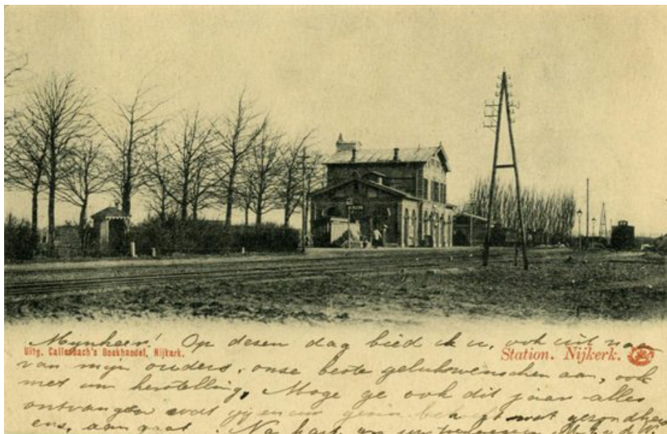
26. Spoorzijde station, 1905. [HUA]
