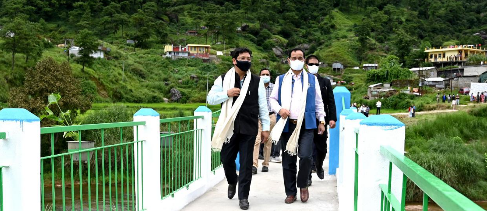
Footbridge over Rilang river at Jashiar (SWKH) constructed under MGNREGS inaugurated by Hon'ble CM and PHE Minister Sh. Renikton Tongkhar
