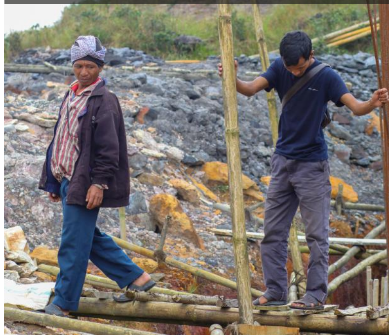
People working under MGNREGS at the Mawrah Bridge, EKH
