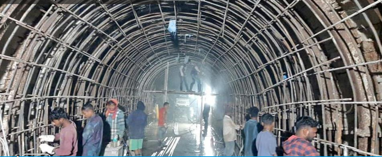
Work at Ganol Hydro Electric Project, West Garo Hills
