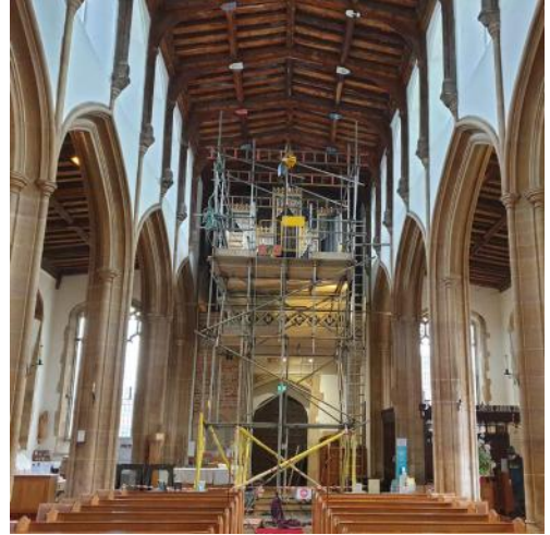
Strengthened scaffolding in place
