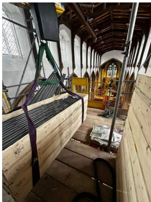
Pipes carefully packed for re-use.
