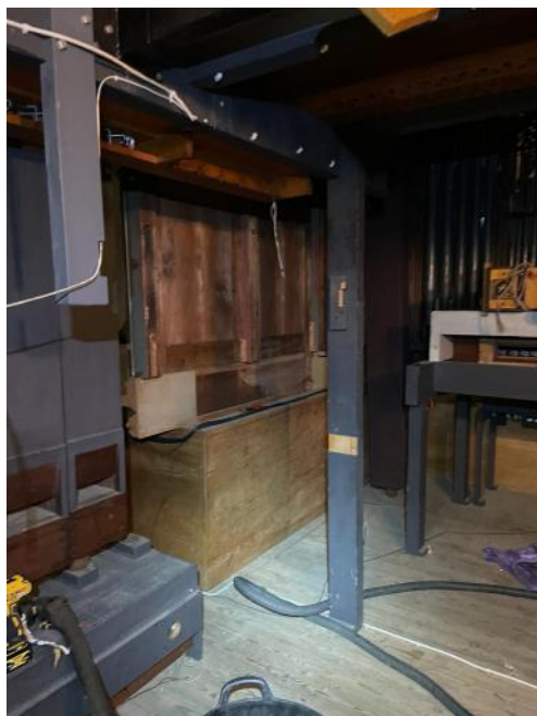
The organ loft partially cleared.
