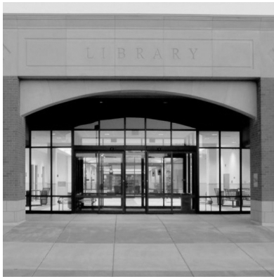
Southwest Library 7979 38th Avenue Kenosha, WI 53142
