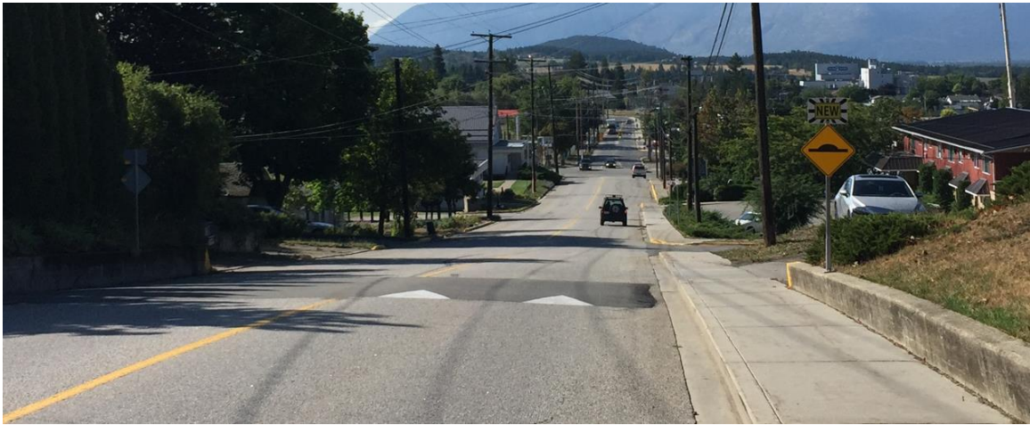
Speed hump on 16th Ave N, near the Creston Valley Hospital
