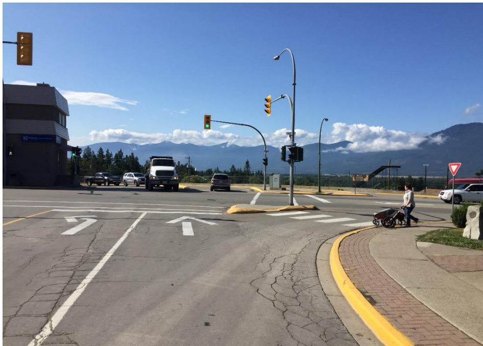
Based on the BC Active Transportation Design Guide, both 16 th Avenue N (top) and 10 th Avenue N (bottom) should be candidates for separated sidewalks.
