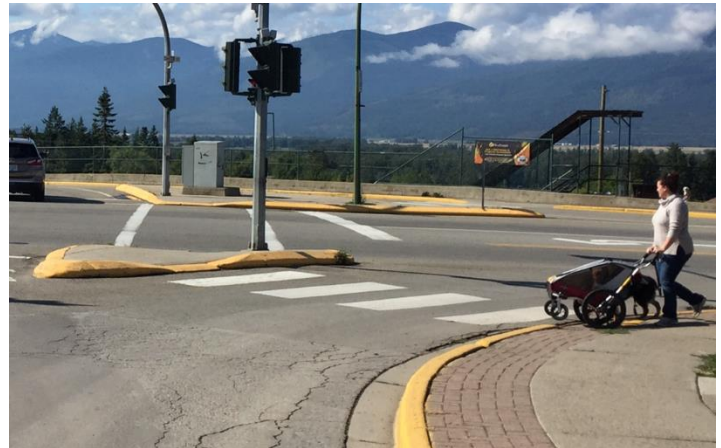
Narrow sidewalk at southeast corner of Canyon Street and Cook Street (left) and poorly designed cut through median / island at the northwest corner (right).
