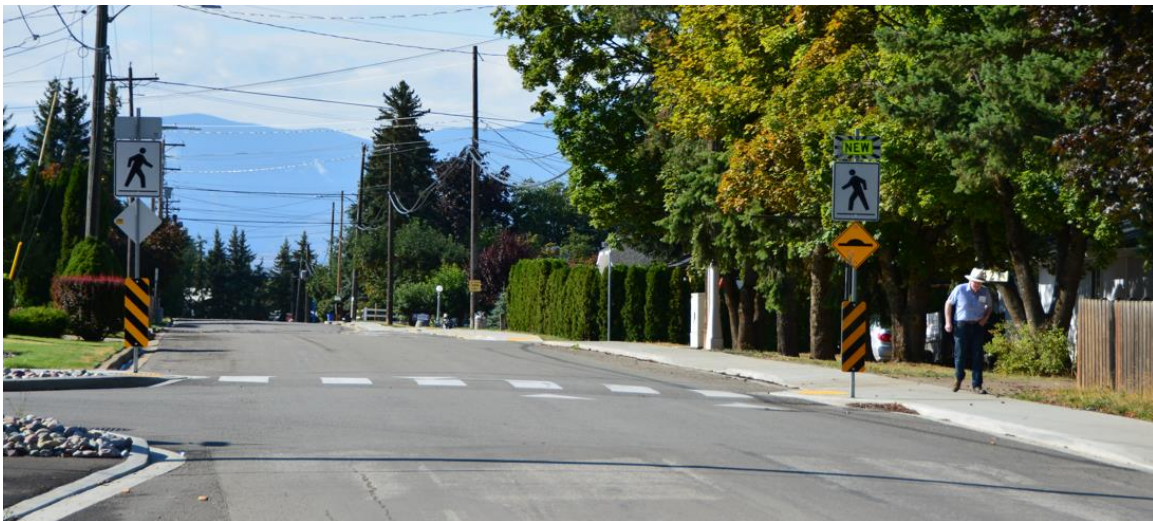
Raised Crosswalk at 20th Ave S and Cedar St
