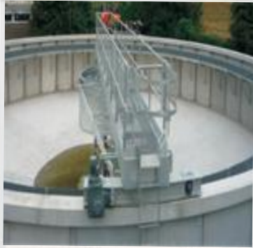
CENTRAL BEARING ASSEMBLY
