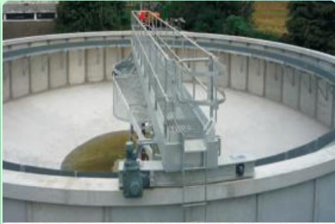
CENTRAL BEARING / CALRIFIER END CARRIAGE DRIVE / FLOCCULATOR DRIVING ARRANGEMENT
