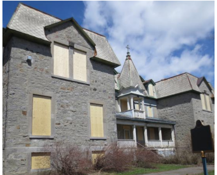
The Bishop's House (boarded up) in April 2015.
