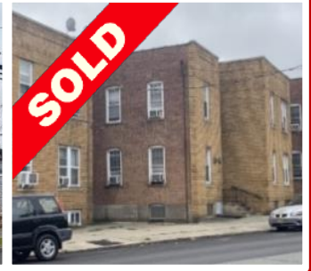
MAIN AVE. PASSAIC
