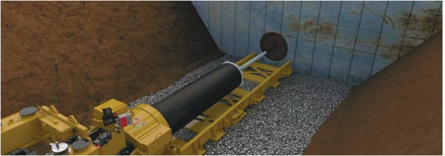
Figure 5: Illustration of starter casing connected to installed pilot tube via a Weld-On Reaming Head (WORH)
