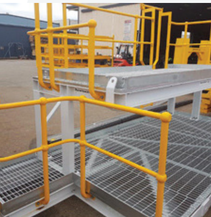
Handrail and Floor Grating
