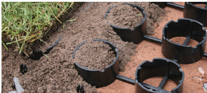
Correct installation of Turf Cells
